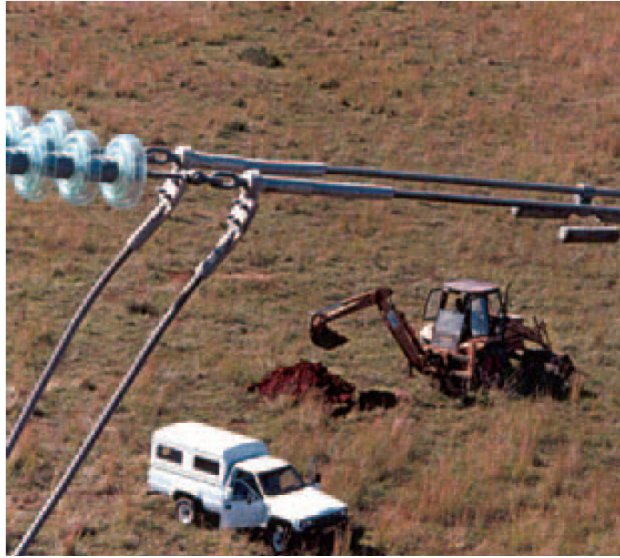
Figure 11.6-1: The construction of a tower foundation.
