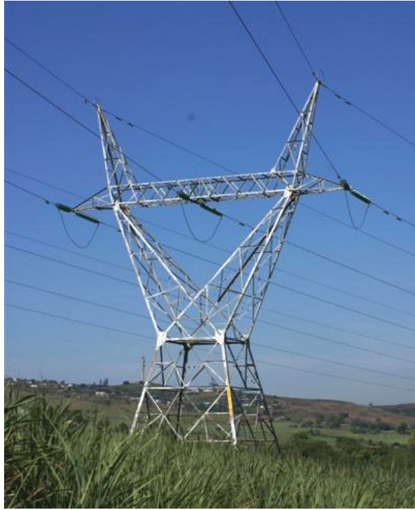
Figure 11.5-10: A typical example of a strain structure
