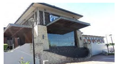
Figure 93 Above : Showing materiality and double volume entrance.
