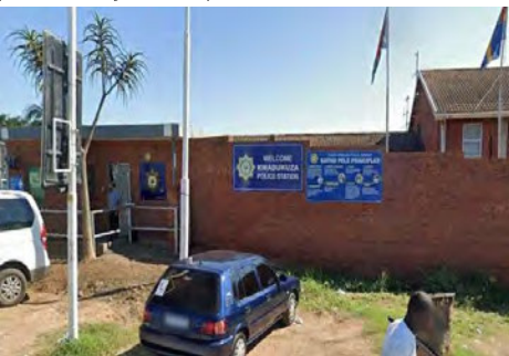
Figure 145 : C: Kwadukuza Police Station - 17 (Source: by author)
