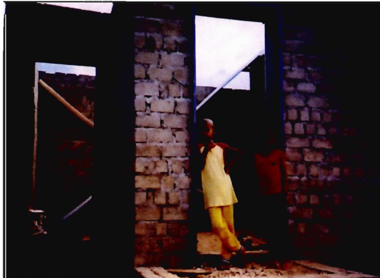
Picture B. Incomplete structure at a roof level.
