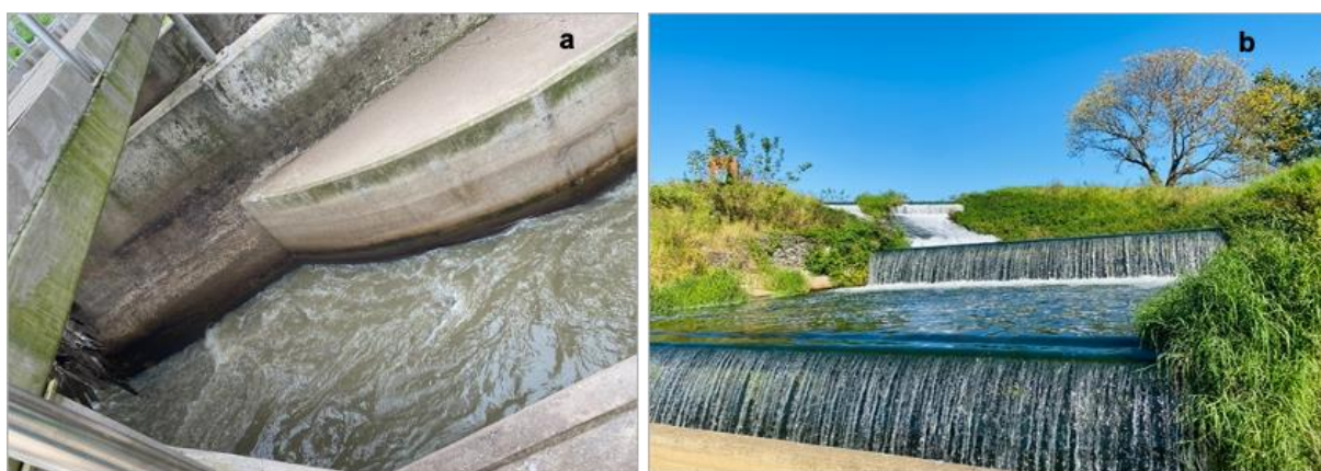
Figure 4.2 Darvill Wastewater Treatment Plant. a = influent and b = effluent
