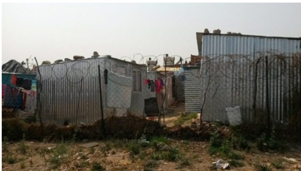
Photo 2: Shacks erected next to Vunani
