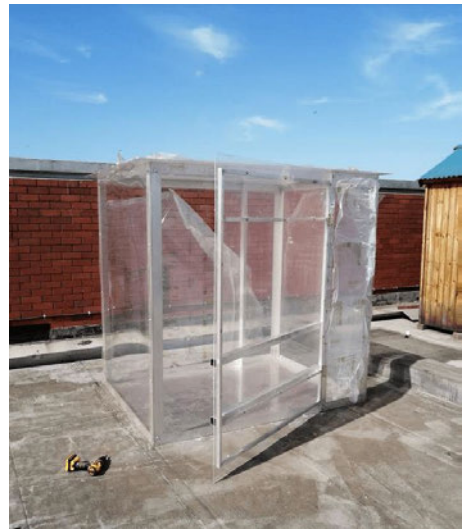
Figure 3-2: Enclosure after its construction.
