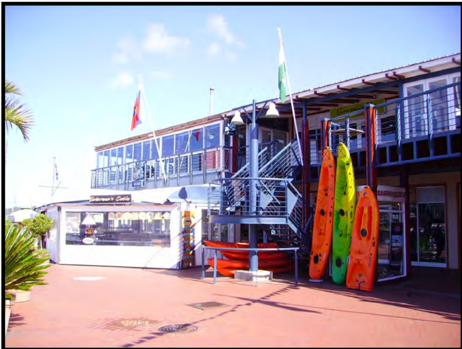
Figure 51 - The small scale of the development is in keeping with the town. It is human scale and fits into its context very well. SOURCE: image taken by author
