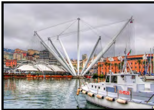
Figure 29 - The Bigo is the new symbol of the regenerated harbour. It is inspired by the derricks that rise from the decks of the cargo ships. Attached to the tallest 'arm' is a type of cable car that gives visitors a bird's eye view of the historic city. SOURCE: www.flickr.com
