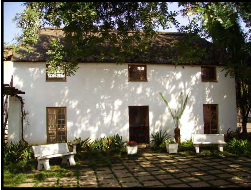
Figure 75 - a circular seating arrangement around a large jacaranda tree provides a contemplative space in which to reflect and dwell on the history and culture experienced at the Msundusi Museum. SOURCE: image taken by author
