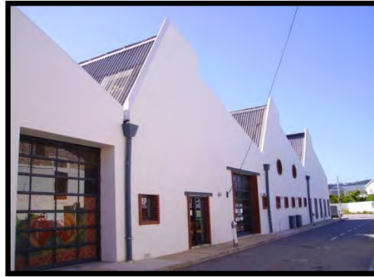
Figure 18 - The eastern wing of the boutique hotel has a new extension that employs the use of modern materials yet shares the same silhouette as the old structure, tying the two together. SOURCE: image taken by author
