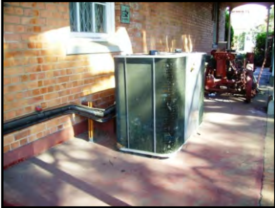
Figure 71 - the old buildings were never designed to store and exhibit valuable artefacts. The buildings in the complex have been retro-fitted with air-conditioning units to keep temperatures and humidity levels low. SOURCE: image taken by author
