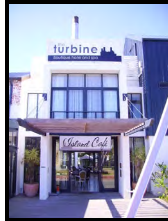
Figure 14 - The side entrance into the Island Café has a combination of old and new materials, effectively showing how the two can successfully mix. SOURCE: image taken by author
