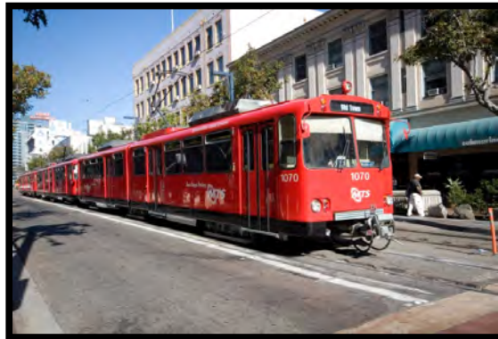
Figure 26 - Smart Transportation: efficient and clean transportation is a major component in developing a sustainable and liveable environment. The San Diego Trolley is both efficient and can transport a large number of people with ease. SOURCE www.upload.wikimedia.org
