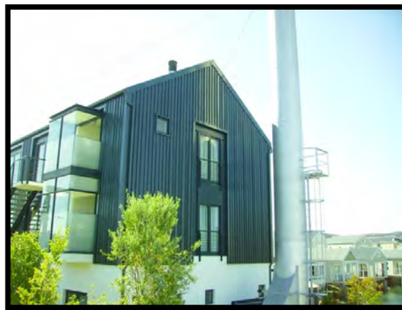
Figure 16 - The eastern wing of the boutique hotel has a new extension that employs the use of modern materials yet shares the same silhouette as the old structure, tying the two together. SOURCE: image taken by author
