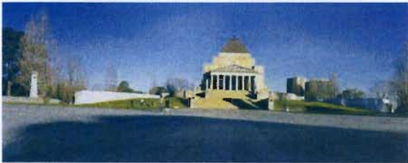
Illustration 57: North Elevation of the Shrine of Remembrance, the new activity is housed in the flanking walls. (Andrew. 2003:52)
