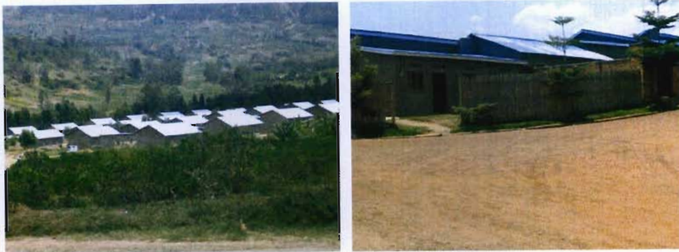
Illustration 68 and 69: shows the housing settlements built for the survivors of genocide in Cyinyinya district (left), and the orphan-headed homes in Kimironko district (right).
