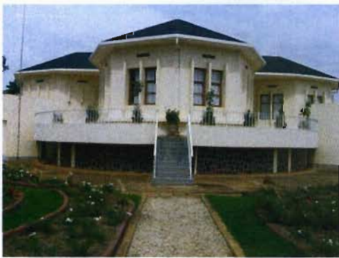
Illustration 74: the exterior elevation of the memorial building showing the domestic-type windows of the memorial.
