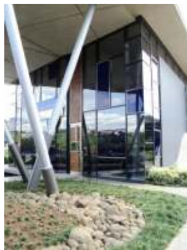
Figure 43. Steel columns and steel frame with structural glass at the entrance (by Author)
