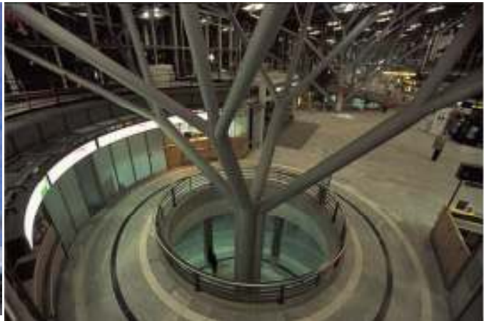
Figure 21. Stuttgart Airport based on the tree branch support system. (Pedersen and Täljsten, 2007:8)
