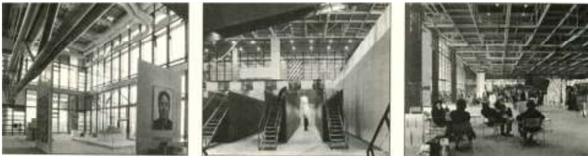
Figure 29. High volumes supported by steel trusses systems enable large panels of glazing and natural light. (Cruiskshank,1997:62)
