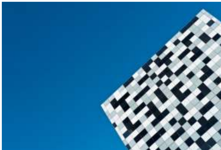
Figure 50. Patterned glazing on the south elevation. (courtesy Paragon Architects)
