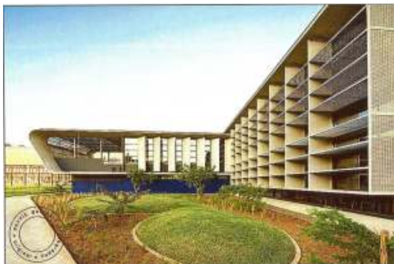
Figure 42. Curved reinforced concrete external structure depicting conveyor belts from the factory(Courtesy EPA Architects)
