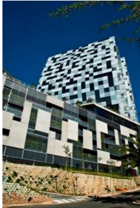
Figure 49. Exterior view of the parking level in comparison to the Norton Rose Towers.
