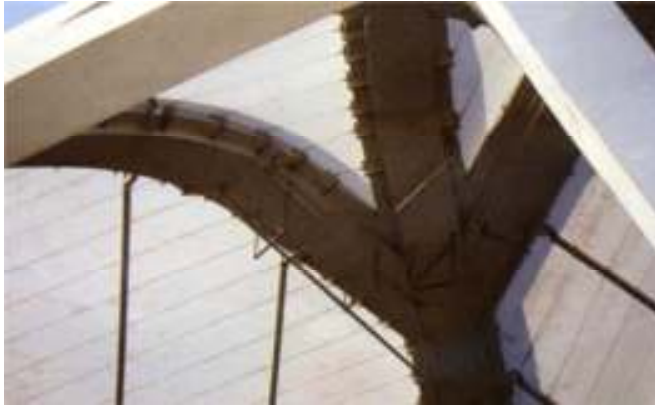
Figure 35. ETFE membrane between steelwork. (Brown, 2009:11)
