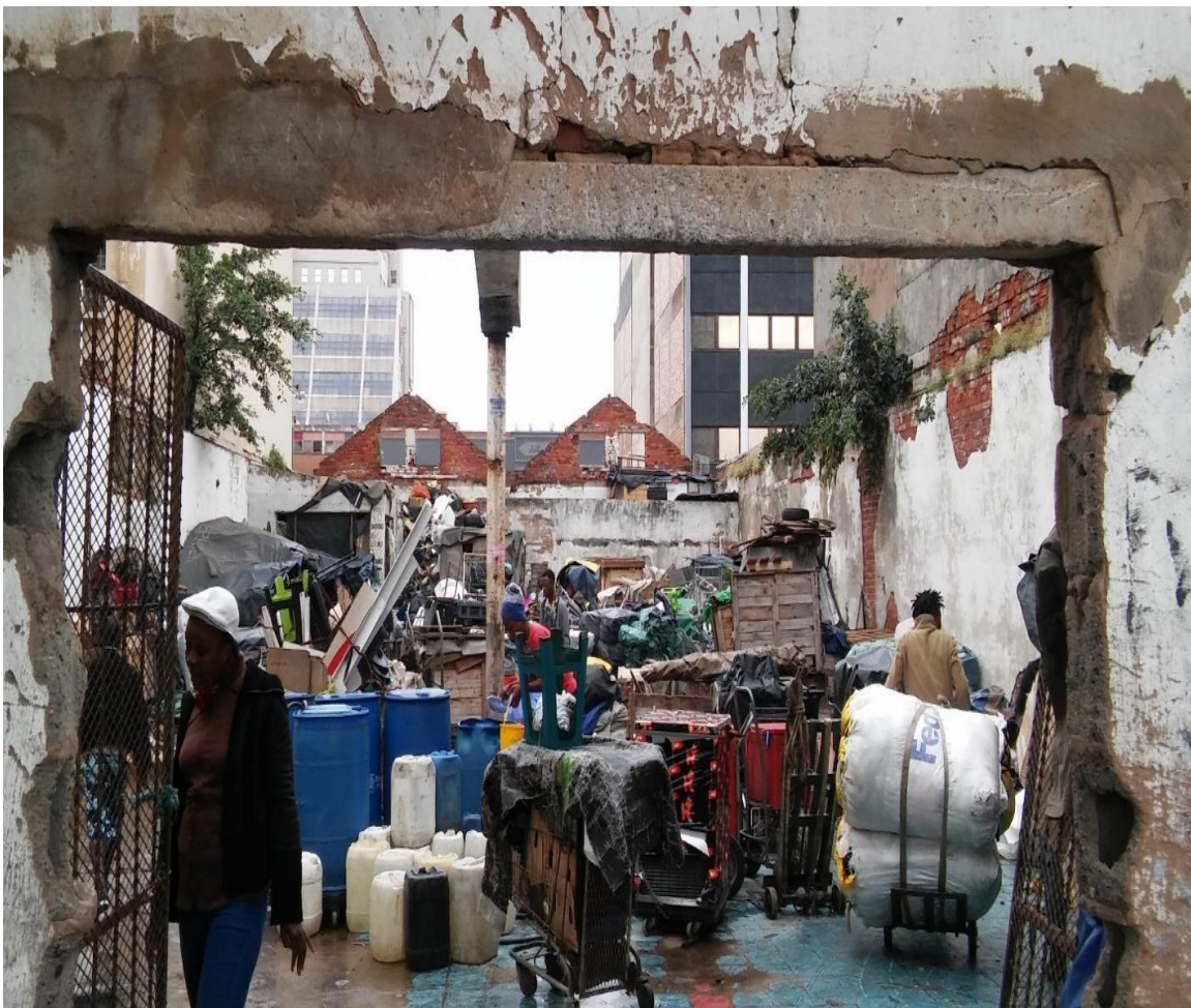
Figure 4.12: Municipality storage facility
