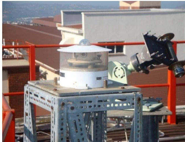
Fig. 2-4 UKZN Westville solar radiometric station. Shown are an Eppley PSP with a ventilation mask and an Eppley NIP.
