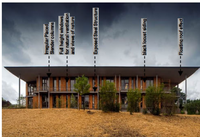
Figure 45. Elevation from Wetlands (Lehoux, 2016)
