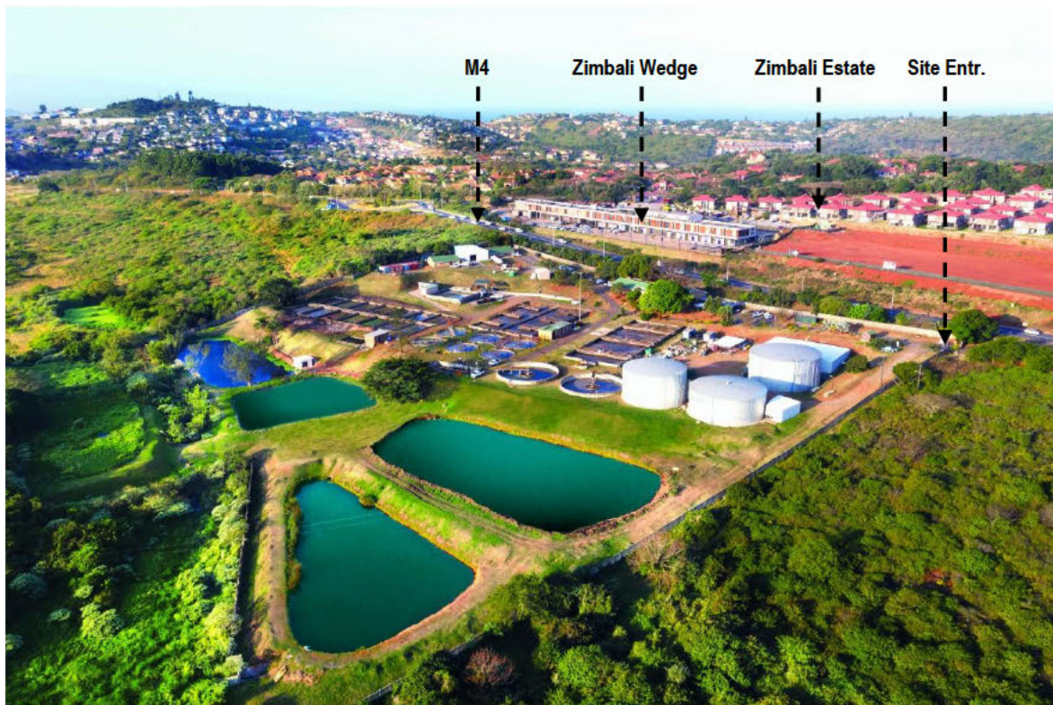
Figure 58. Overall View of the Recycling Plant (Siza Water, 2021)
