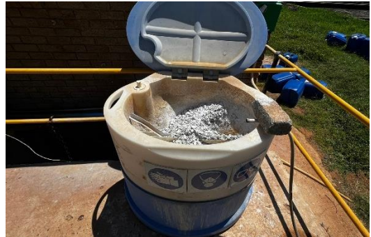
Figure 64. Chlorine Chips (Author, 2023)
