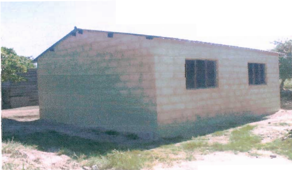
Plate 6: A modern structure of the subsidy housing
