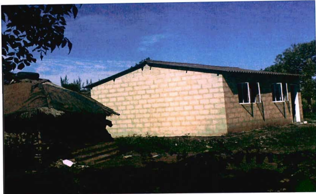
Plate 7: Subsidy Housing in Mpukunyoni area
