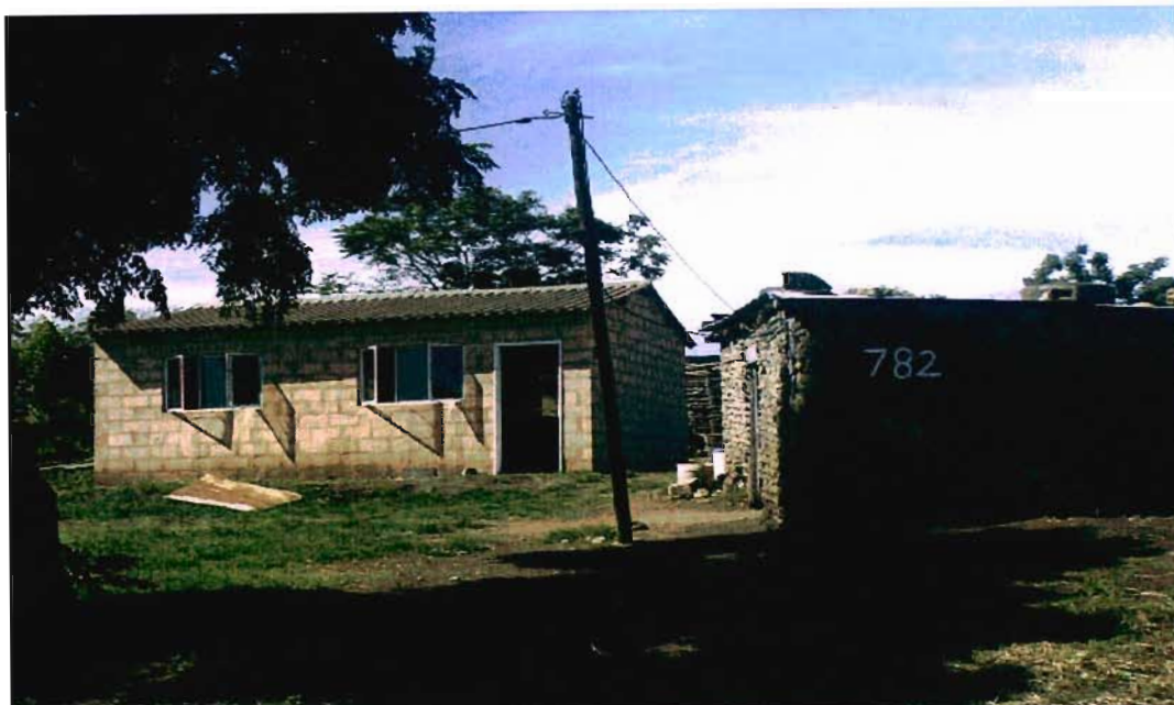
Plate 8: Subsidy Housing in Mpukunyoni area
