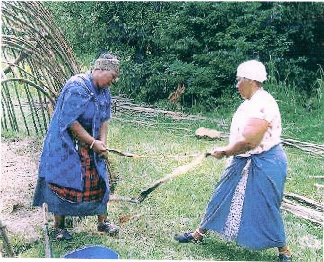
Plate 1: Beehive under construction
