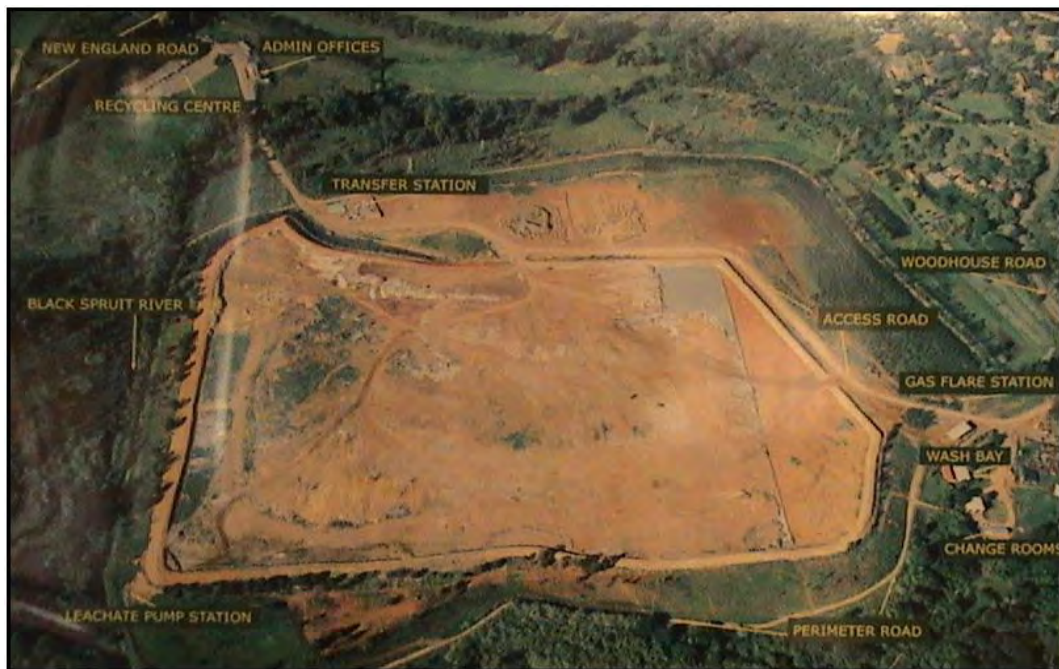
Figure 7.2 – Aerial view of the New England landfill site (Source: uMgungundlovu District Municipality, 2010)
