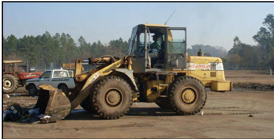
Figure 8.6 – Waste removal from demarcated work area after sampling
