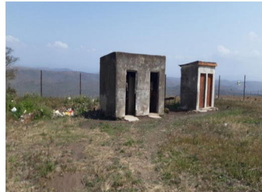
Figure 2.14: Ablution facility in the North Coast Region of KwaZulu-Natal (Author s Observations)
