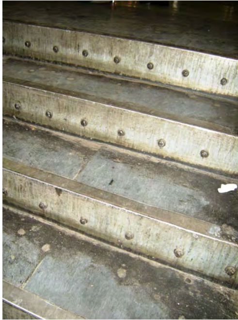
Figure 5.12- Protected edge detail on staircase. (Author)
