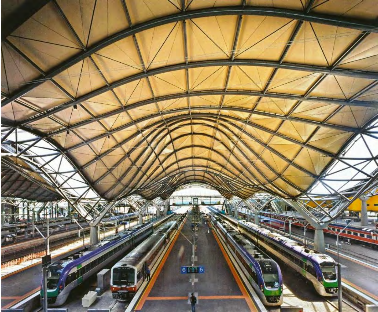
Figure 4.17- An image showing the typical bay of the roof structure. Columns are designed to intersect every second platform to maximise flexibility (Grimshaw, 2008: 799)
