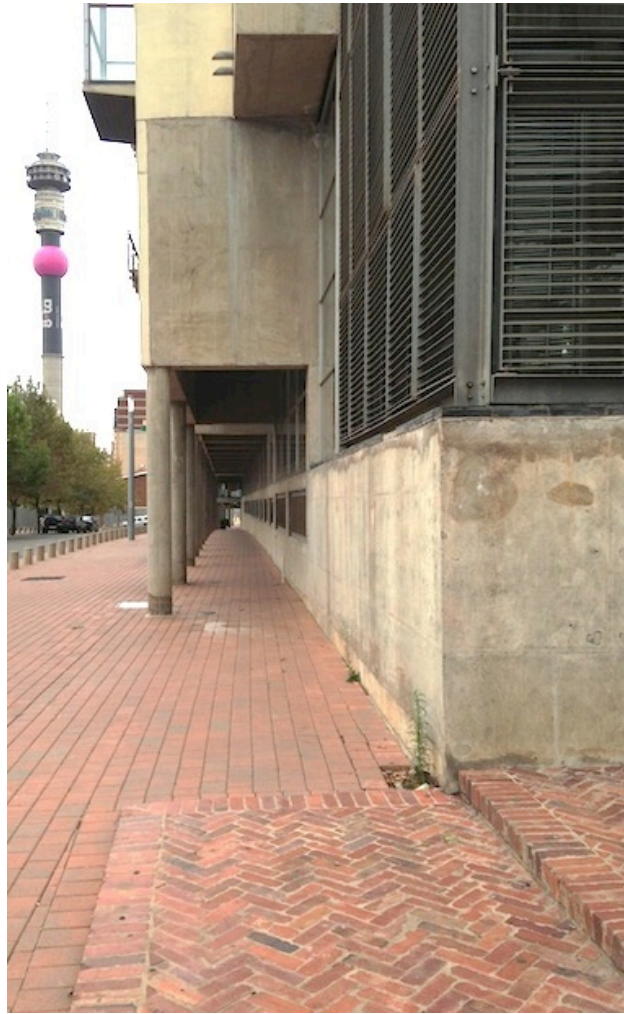
Figure 73 Main materials used are clay brick, steel and concrete in various finishes. Source: Author
