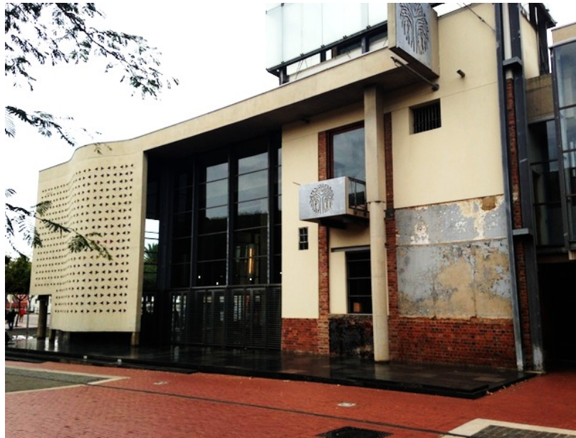
Figure 76 The south facade with fully large curtain walls. Source: Author
