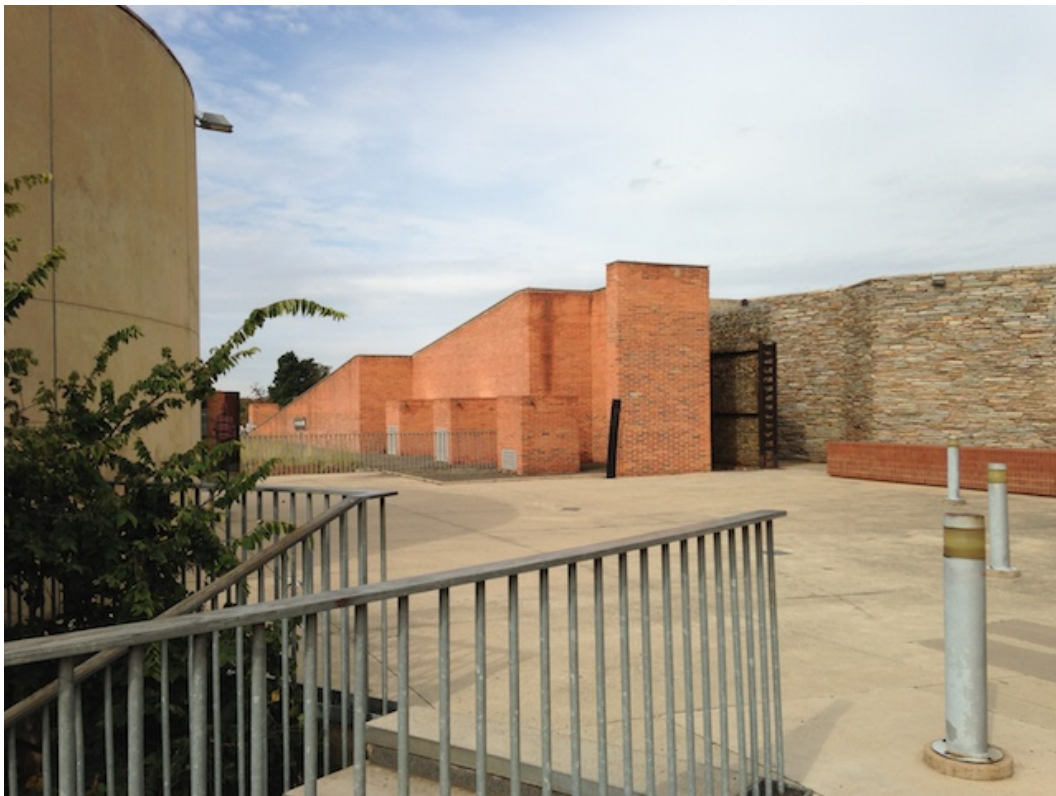
Figure 58 High walls screening the surrounding theme park and casino. Source: Author
