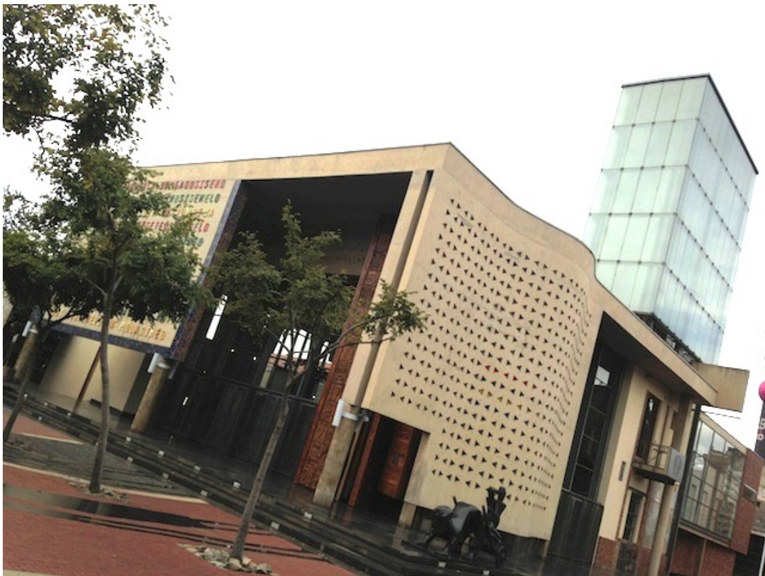
Figure 85 The glass tower over the foyer representing the highest point of the building over its most important communal space. Source: Author
