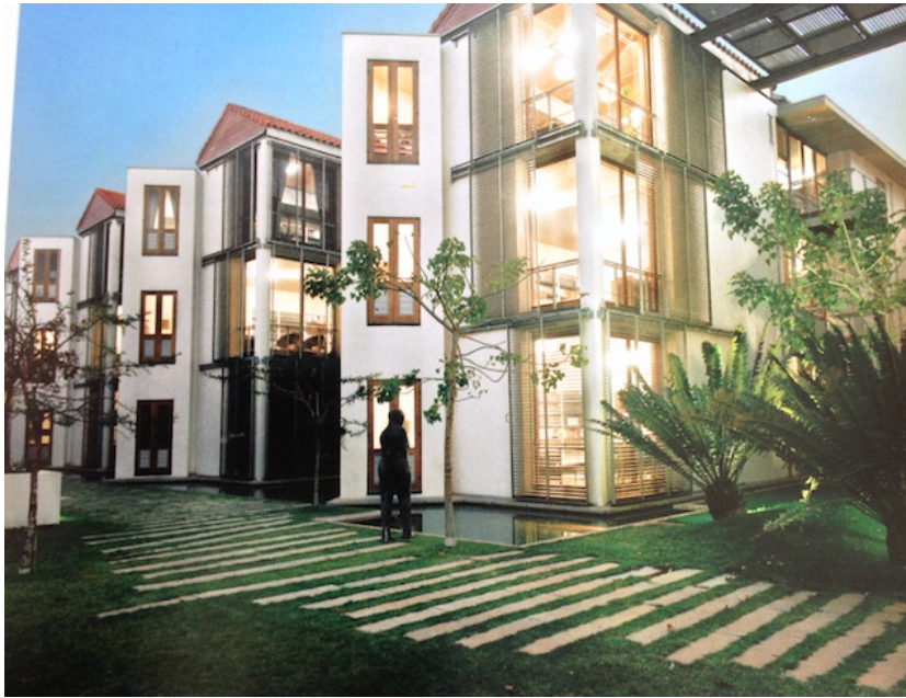
Figure 77 The justices' offices overlooking the inner courtyard. Source: Law-Viljoen, 2006: 117.
