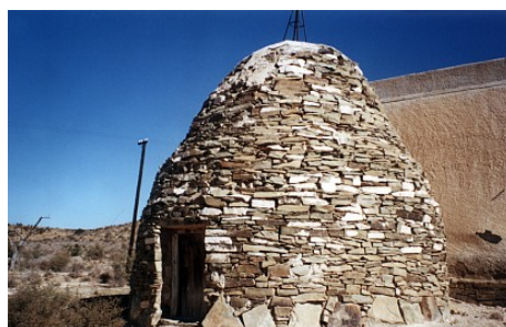
Figure 54 Corbelled parabolic stone dome by the 19th century settlers in the Karoo. Source: Malan and McInerney, 2001: 75.
