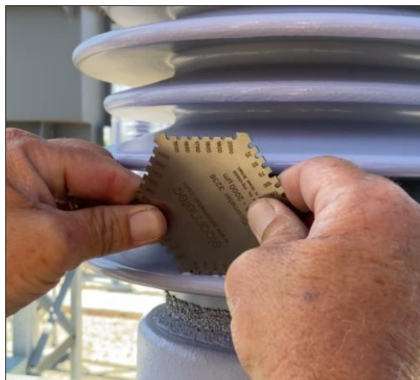
Figure 13: RTV SR wet film comb thickness measurement observation at a coastal substation near Cape Town.
