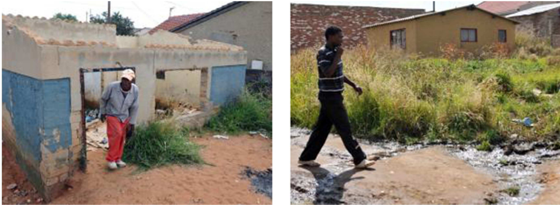
Figure 2-12: The RDP settlement at Braamfischerville. (Source: IOL, 2012)
