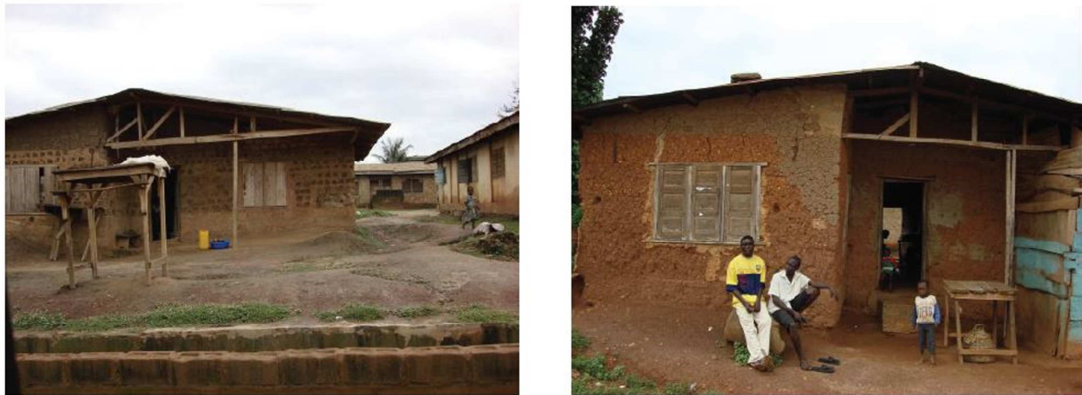
Figure 2-16: Low-income housing in Ogebere, Nigeria. (Source: Jaiyeoba & Aklanoglu, 2012)
