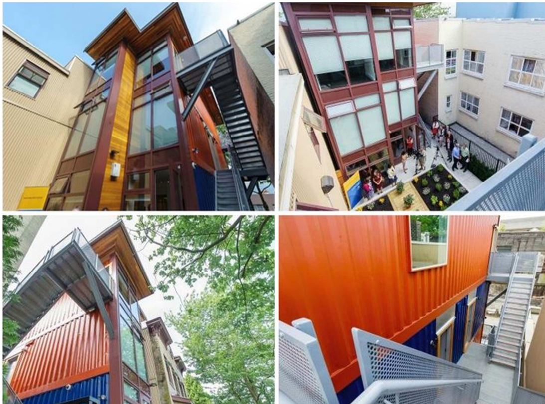
Figure 2-28: First containers social-housing in Canada. (Source: Atira, 2013)
