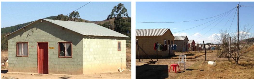
Figure 5-8: Views of the RDP units in Bulwer
