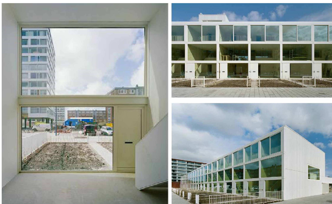
Figure 2-25: Town Houses social housing, Amsterdam. (Source: Atelier Kempte Thill, 2008)
