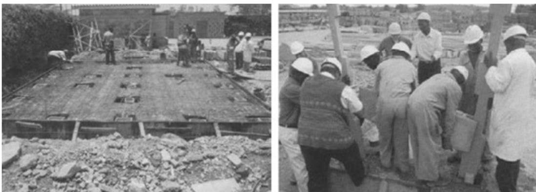
Figure 2-20: Roofing, Pumwani, Kenya. (Source: Shitote et al. , 2006)
