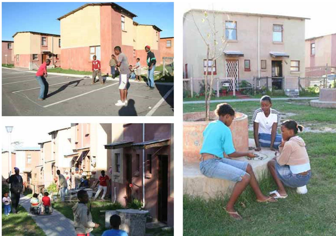
Figure 2-11: Sakhasonke Village. (Source: Impulelelo Municipality, 2006)
