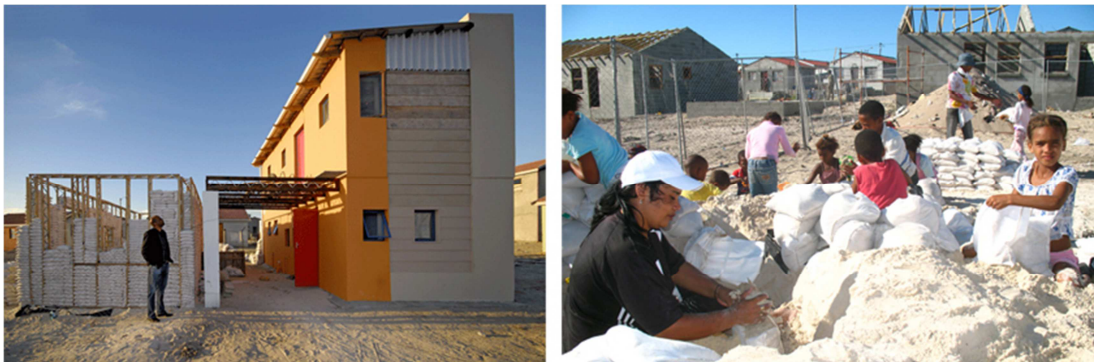
Figure 2-10: Views of the 10x10 housing project in Freedom Park. (Source: Design Indaba, 2008)
