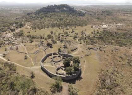
PLATE 4.3.3. Ariel view of Great Zimbabwe. (Source: Google).
