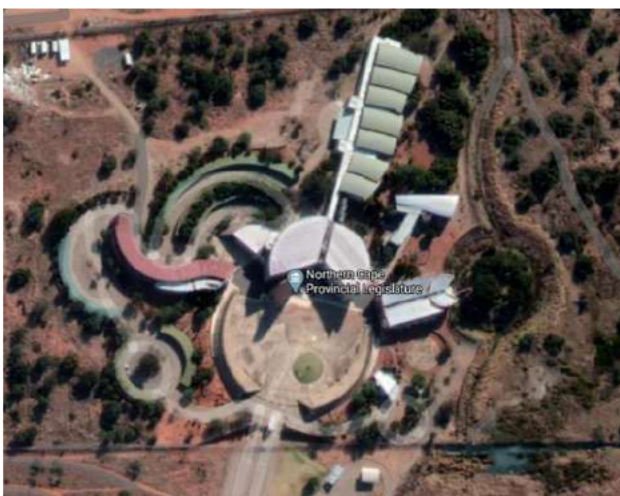
PLATE 5.3.5. Northern cape Legislature building site
