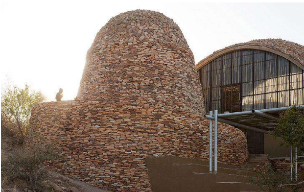
PLATE 5.2.9. View showing Undulating vaults bear lightly on the side walls and Glass panels (Archdaily search. Accessed 23/10/2019).
