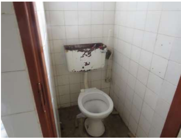
PLATE 6.2.34. female Toilet cubicle . ( Source: Author).
