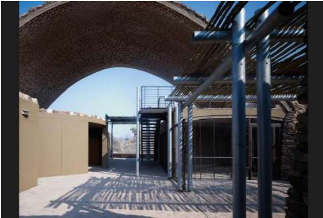
PLATE 5 2 8. External terraces shaded by horizontal slats to create areas reminiscent of the traditional African gathering space, or kgotla. (Archdaily search. Accessed 23/10/2019).
