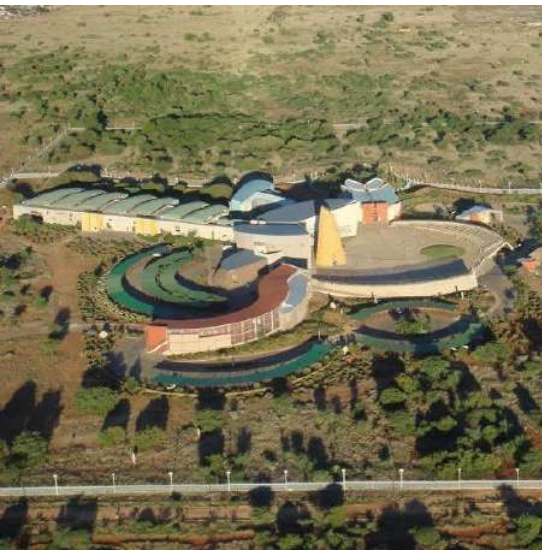
PLATE 5.3.8. Outer walls as you approach the Legislature are in the shape of buffalo horns protecting the kraal. (Google search. Accessed 23/10/2019).
