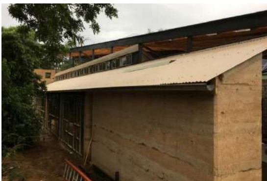
PLATE 5.4.8. Breathable, fireproof rammed earth wall
