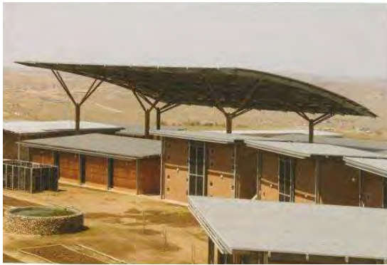
Fig 2. 8- Main canopy providing protection to the single storey buildings below (Eicker, 2007; 20).
