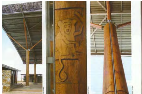
Fig 2. 9- The main canopy's columns are steel clad in timber to symbolise the forest (Eicker, 2007; 21).
