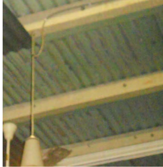
Fig 4. 7- View of internal roof structure with exposed materials (By Author).
