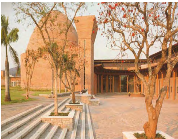
Fig 4.16- The Square at the Legislature which is the primary space for gatherings (Malan, 2001; 40).
