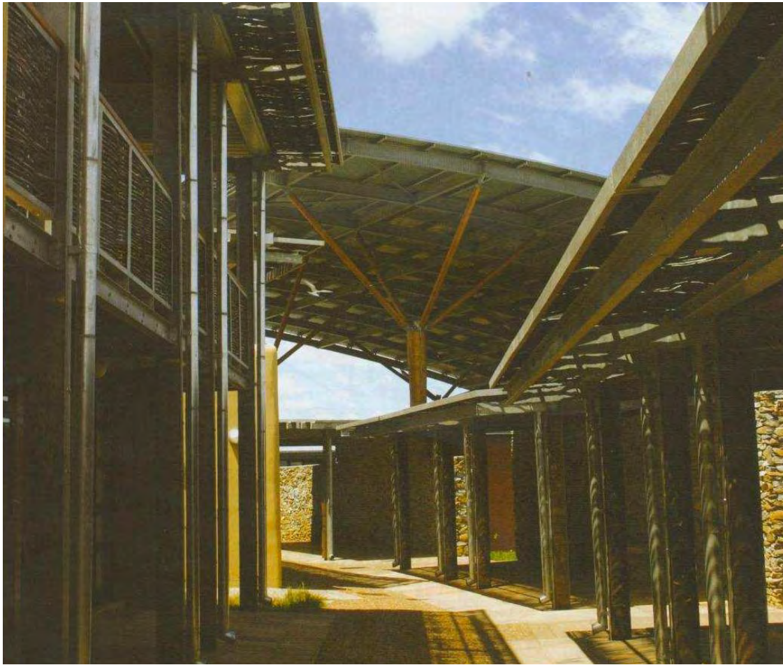
Fig 2. 10- Image of Village street between buildings which forms an open thread through the centre (Eicker, 2007; 16).
