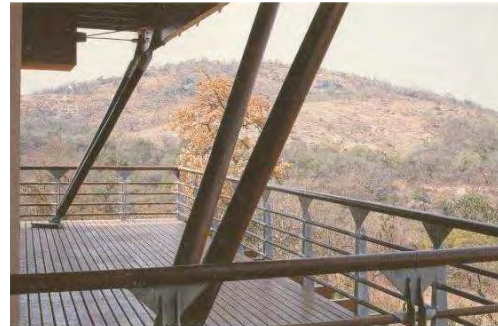
Fig 4.13- Eastern edge of complex which interacts with nature and provides views of the landscape (Malan, 2001; 32).
