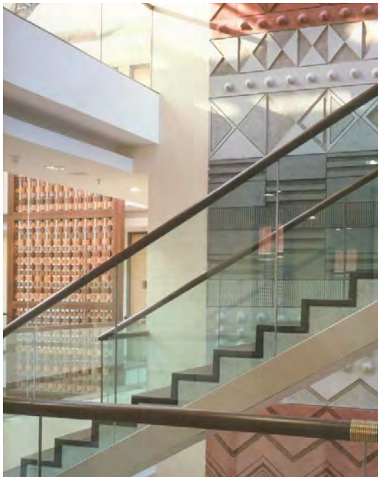
Fig 2.25- Coloured and textured sculptural plaster finishes on walls ('Architect and Builder', 2004; 29).
