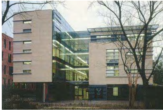
Fig 2.23- Sandstone cladding used at front facade ('Architect and Builder', 2004; 20).
