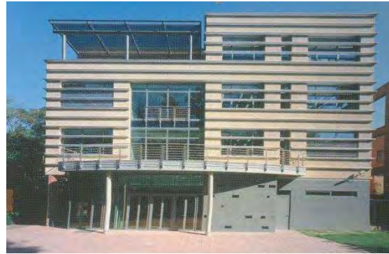
Fig 2.24- Rear facade highlighting horizontal aluminium elements ('Architect and Builder', 2004; 22).
