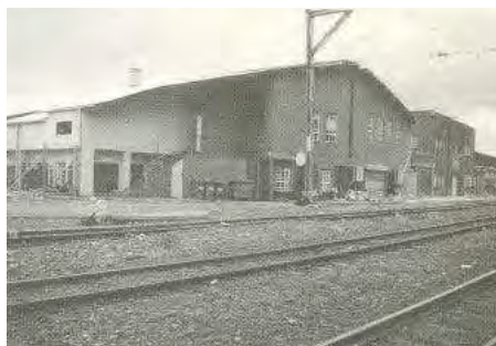
Fig 4. 3- North elevation of BAT Centre with railway line barrier (Claude, 1996; 6).
