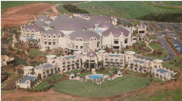
Fig 2.30- Sibaya Casino and entertainment complex showing details with elements reminiscent of royal Zulu crowns, which can also be viewed as a collection of izicholo (plural for isicholo). The circular forms could also be seen to represent a collection
