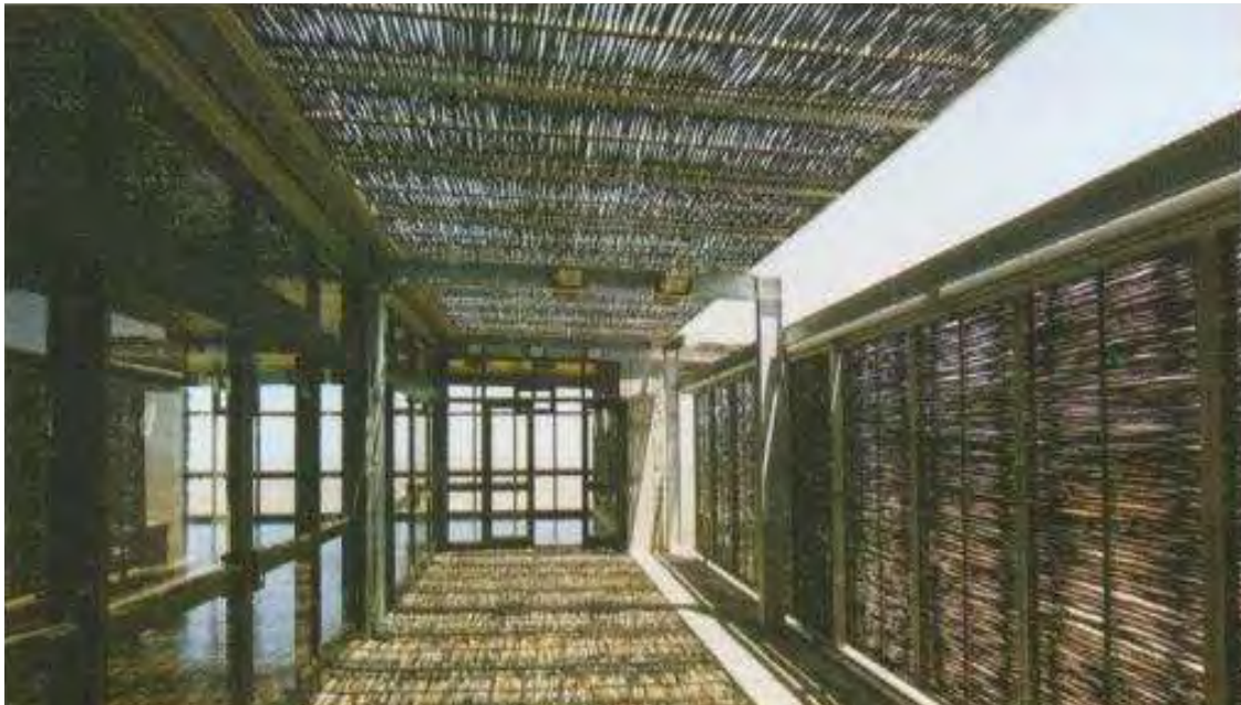
Fig 2. 7- Latte screens used as shading devices and as a means of privacy and the screens were made from locally harvested wattle branches (Eicker, 2007; 18).
