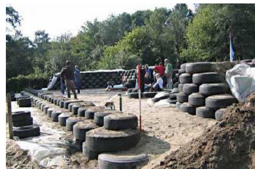
Figure 1.23: Earth-packed used tyres as walls. Labour intensive and time consuming (Source: URL95).
