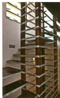
Figure 1.16: Ad hoc staircase – bolted connections (Walton, 2011).
