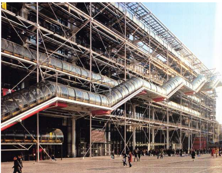
Figure 2.10: Centre Pompidou in Paris. The “externalised skeleton” supports large spans which render the interior rooms extremely flexible – there are no internal supports, hence the notion of an “open structure” (Gössel et al , 2005: 458).
