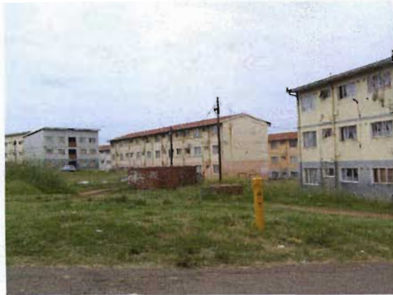
Illustration 90, Reiger Road flats popularly known as "Destroyer flats" erected by the Department of Community Development
