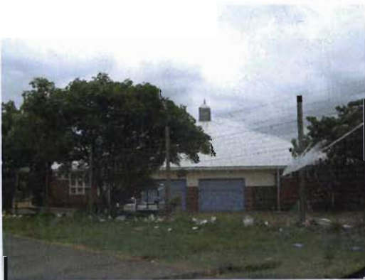
Illustration 100, The community hall and surrounds
