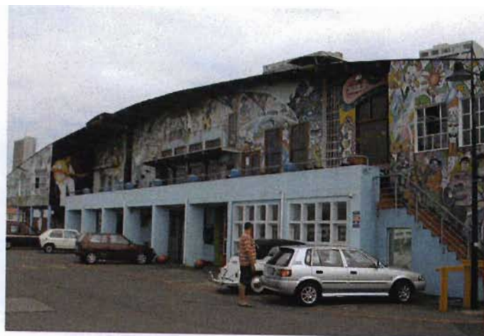
Illustration 52, View of the curved corrugated iron roof
