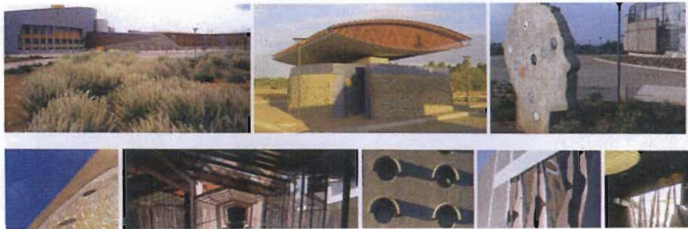
Illustration 16, Legislature for the Northern Cape Provincial Government, showing the local artwork, landscape and detailing of the building
