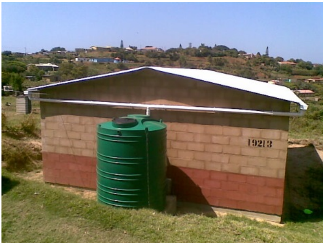
Plate 3: UMzumbe- Turton low-income housing water storage
