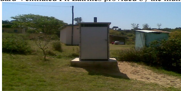
Plate 4: RDP standard Ventilated Pit Latrines provided by the municipality
