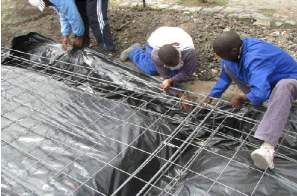
Figure: 2 Youth building houses
