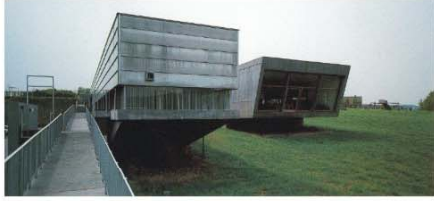
Illus. 22- the approach ramp from the bottom of the site. (Quadrants No.214, 1996/102)
