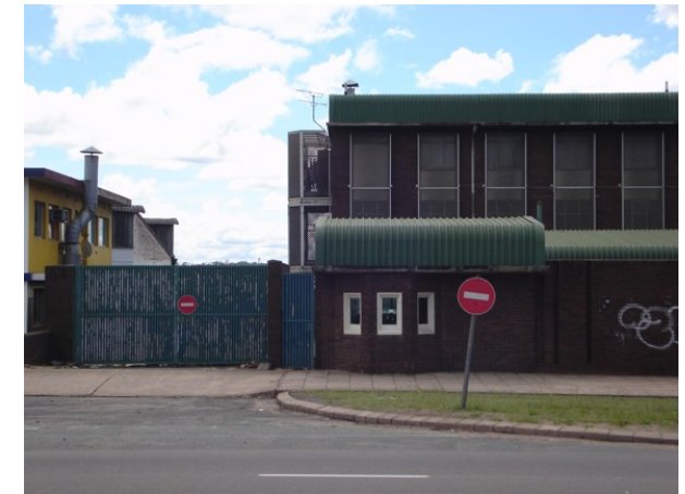
Illus. 2- Pinetown Police Station, an SAP Fortress. (Note Screens over windows and defensive measure at entry point)
