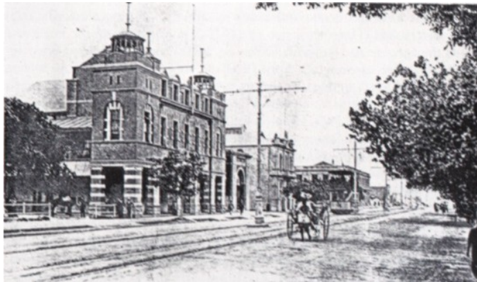
West Str Police Strn in early 1900's.Colonnaded entrance and towers at each end, one of which housed the curfew-bell that signaled 'natives' having to be off the streets by 21h00. (Jewel, 1989: 12)
