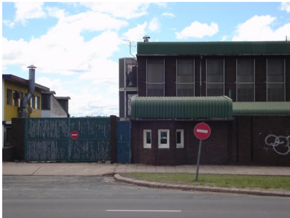
Illus. 53- The non-functioning police entrance.
