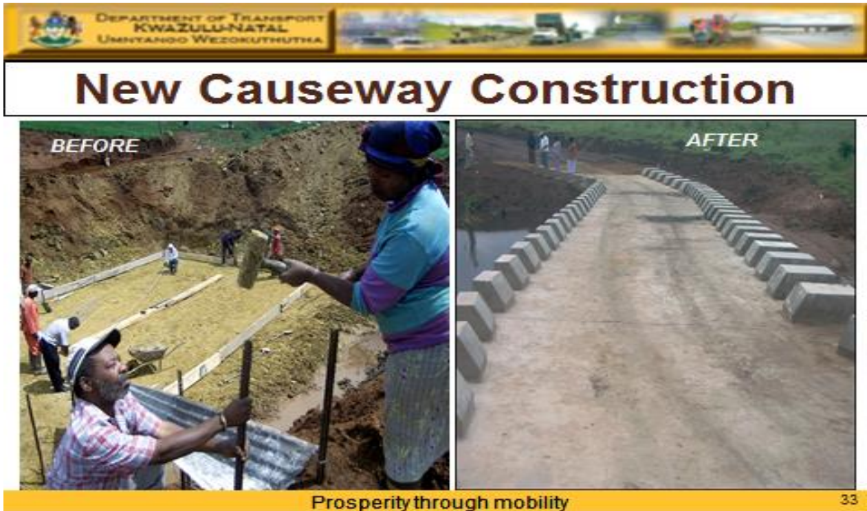
Figure 1.1: Bridge construction by Vukuzakhe Contractor (KZN DOT, 2015a).
