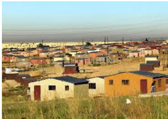
Figure 4: The developing side of Mthwalo.
