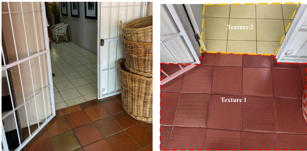
Figure 6.8 depicts the change in texture that has similar properties and therefore does not offer much clarity on the differences for the visually impaired. (Source: Author, 2022)
