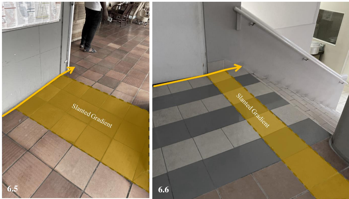
Figure 6.5 and 6.6 Show how topographical changes are used as cues on thresholds to communicate about the spatial characteristics in the building. (Source: Author, 2022)
