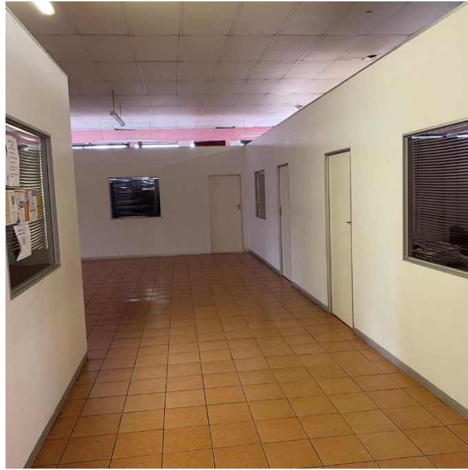
Figure 6.12 shows how monotone colour surfaces make it more difficult for the visually impaired to spot the fields of interests such as doors on the walls. (Source: Author, 2022)
