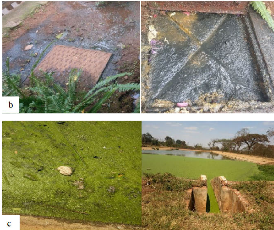
Figure 2.2 Field examples of the causes of failures in the sanitation value chain (Photos taken by the author)
