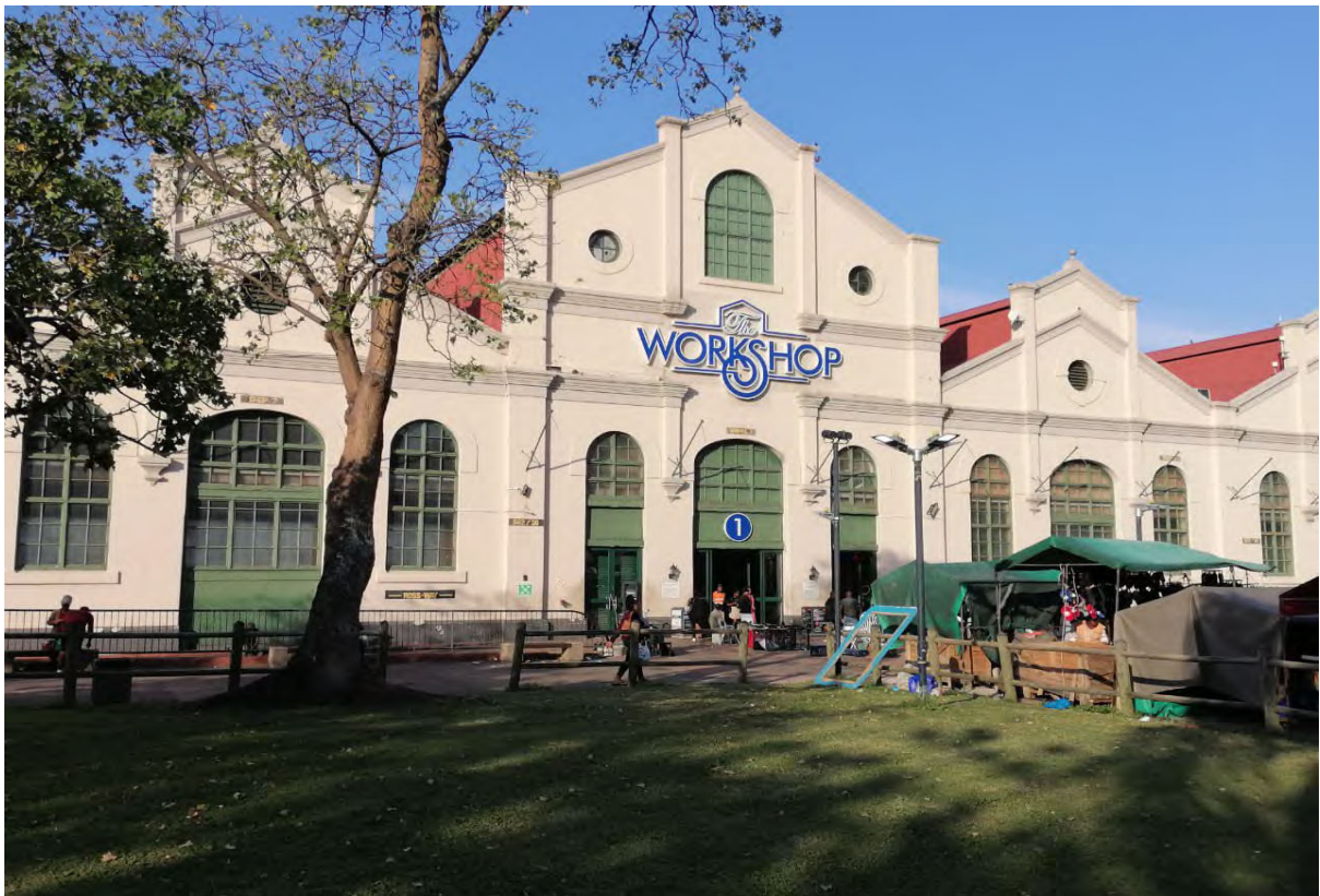
Figure 4.3: Durban CBD Workshop
