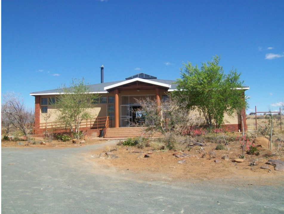
Image A1: The front façade of Wildebeest Kuil. Source: Barnabas, September 2012.
