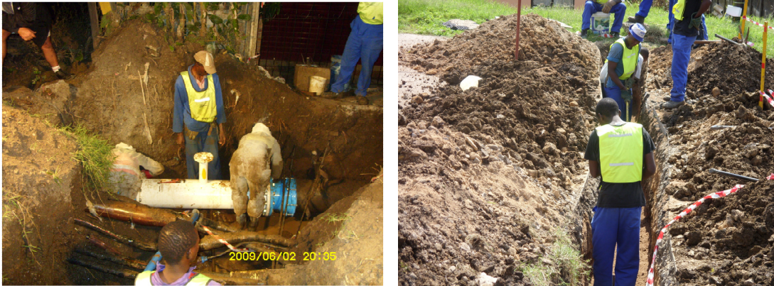
Photographs 1 & 2: Learners working on water projects
