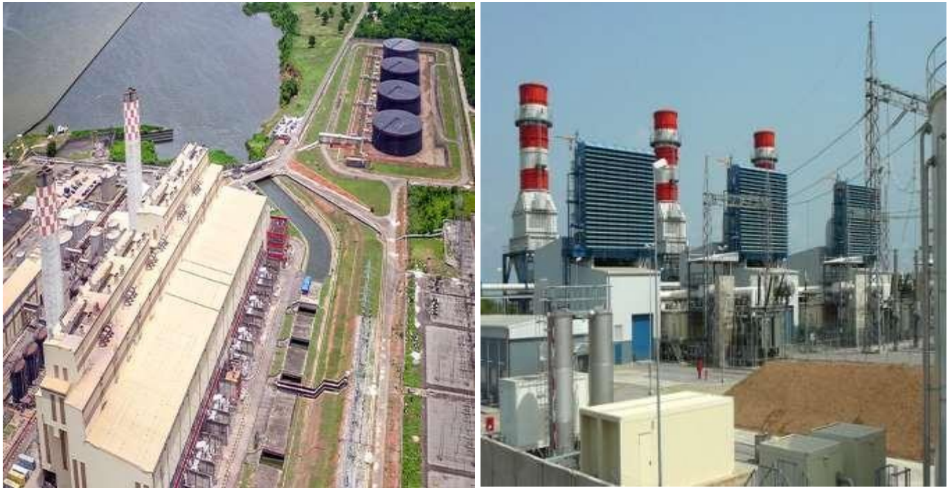
Figure 3.9: The Egbin Power Plant
