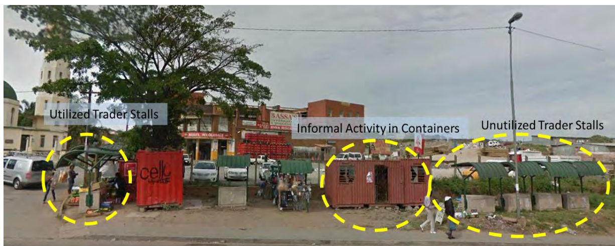
FIGURE 39: IMAGE SHOWING UTILIZED AND UNUTILIZED INFORMAL TRADER STALLS WITHIN THE WIGGINS/BELLAIR NODE
