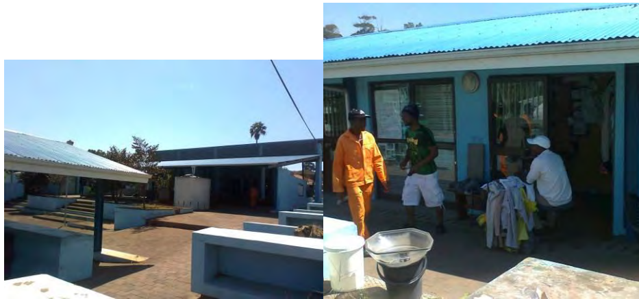
FIGURE 38: IMAGES SHOWING INSIDE OF THE MARKET FACILITY (SOURCE: AUTHOR, 2014)
