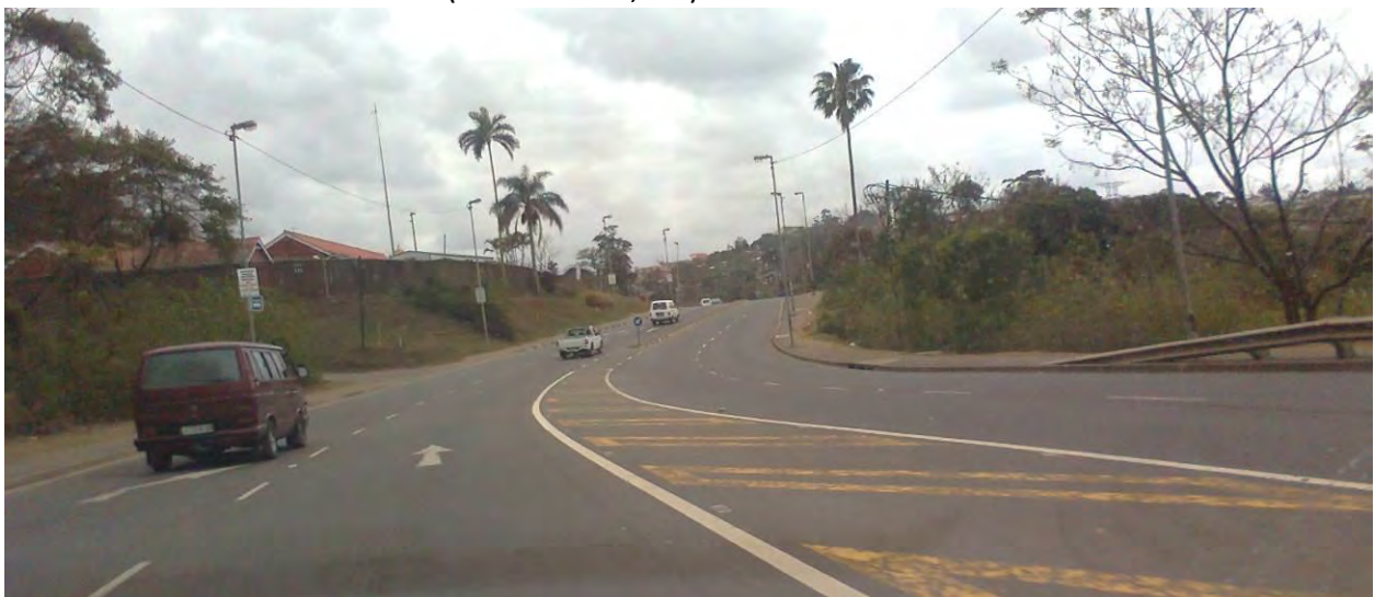
FIGURE 15: IMAGE SHOWING ROAD RESERVE (SOURCE: AUTHOR, 2012)
