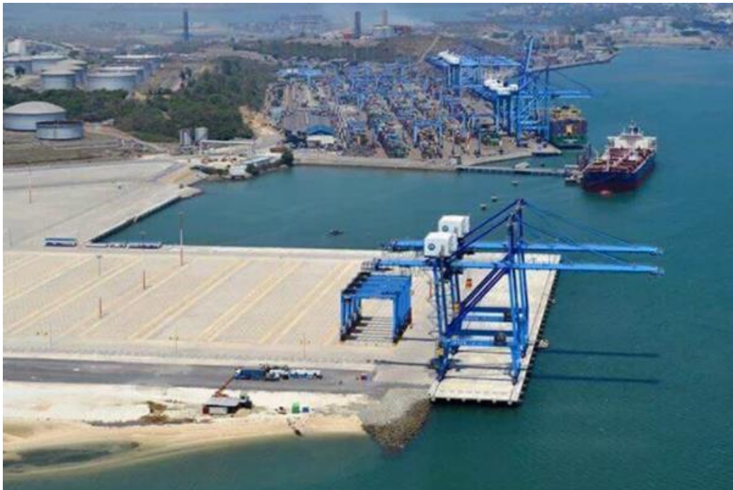
Image 5.3 New container terminal under construction at Mombasa
