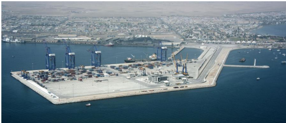
Image 5.4 New container terminal at Walvis Bay
