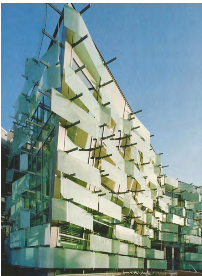
Figure 71 The broken façade (source: Berg 2009: 62)
