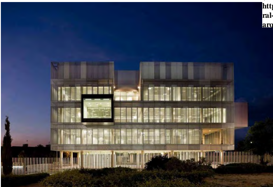
Figure 85 The light shines through the mesh at night v=creating a beacon of light and a symbol of safety (source: http://www.archdaily.com/255186/fuencarral-el-pardo-police-station-voluar-arquitectura )
