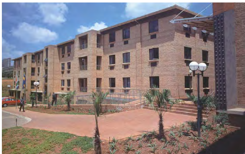
Figure 58 The facebrick façade of the SAPS headquarters (source Gauteng Provincial Headquarters for SAPS. 2004: 75)
