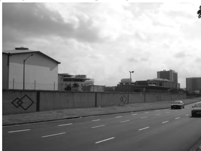
Figure 21 Site B is the existing old fort substation which is to be relocated (source: author)
