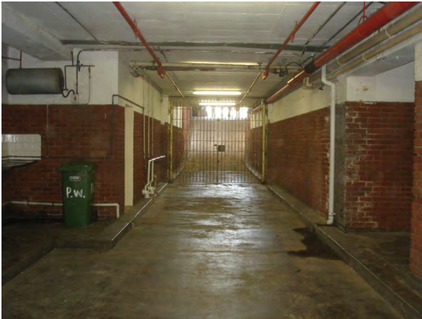
Figure 46. Prisoner's entrance into the basement (source: author).
