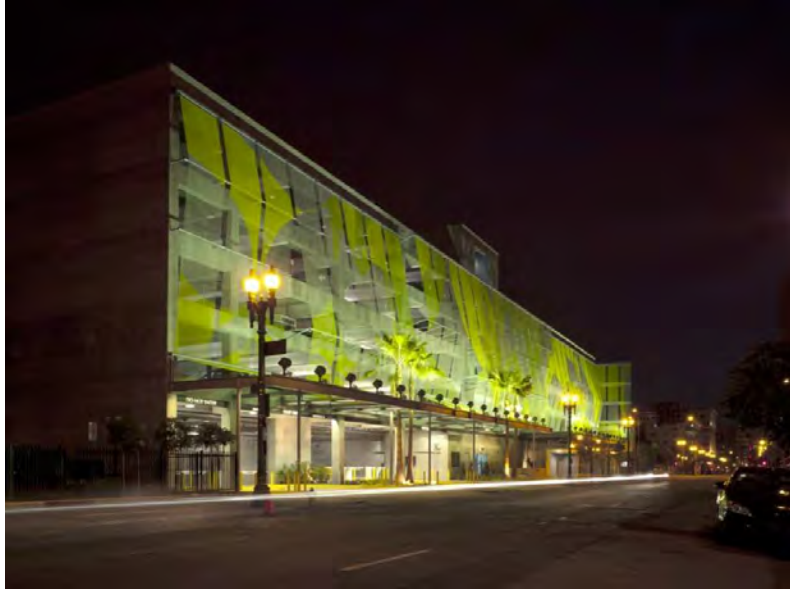
Figure 81 The stainless steel mesh allows an ever-changing façade which appears to glow at night. It also gives the building an interesting play on transparency (source: www.archdaily.com/139804/lapd-mtd-msp-john-friedman-alice-kimm-architects )
