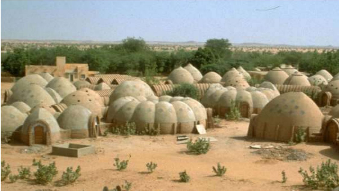
Figure 17: Fabrizio Carola hospital in Kaedi, Mauritania amalgamated traditional and modern construction methods (Derakhshani, 2012:32).
