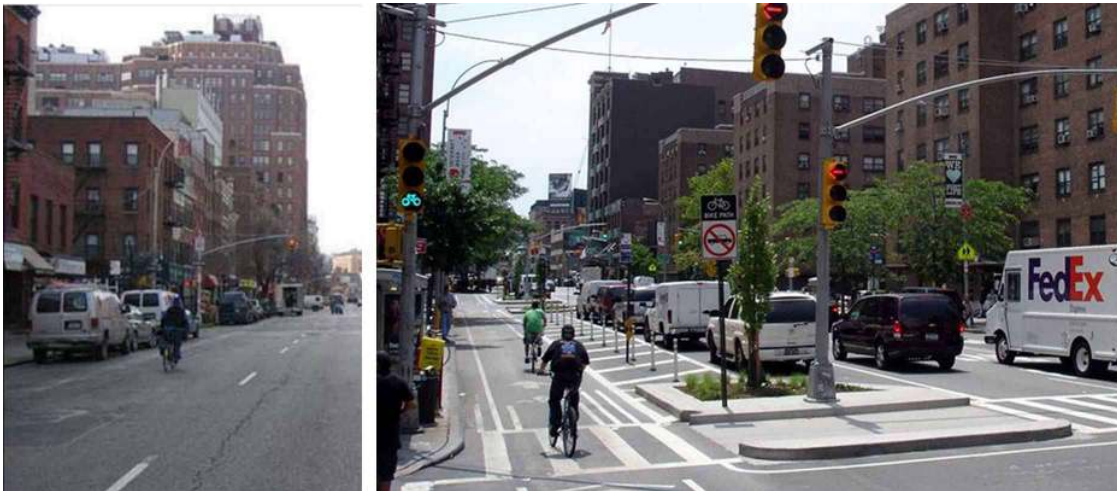
Figure 8: 9th Avenue, Manhattan before (left) and after (right) a 2008 "Copenhagen style" bicycle path designed, so that parked cars protect bicycle traffic. Bicycle traffic has since doubled in New York, in only two years (Gehl 2010:11).
