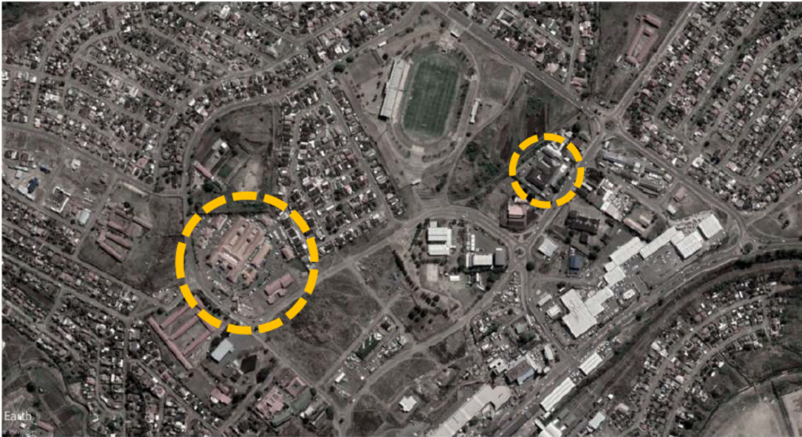
Figure 42: KwaMashu Community Health Centre (left) together with KwaMashu Poly Clinic (right) which it replaced in 2011 ( www.google.com/earth ).
