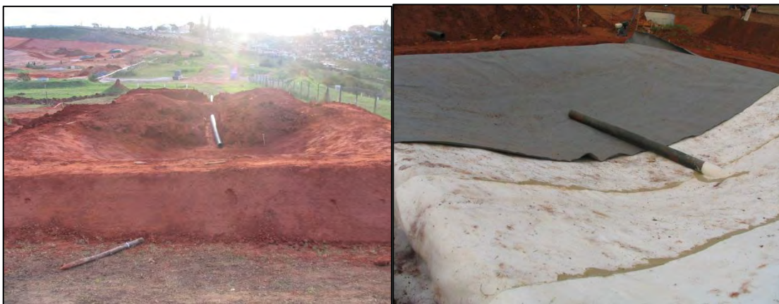
Figure 2.8-3: Construction of cell walls and installation of GCL and protective (Simelane, 2007)
