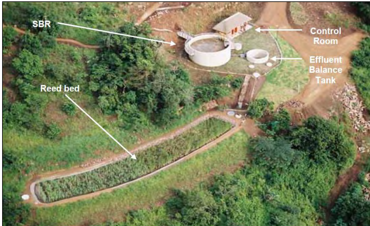
Figure 2.8-2: Aerial view of Mariannahill Leachate Treatment Plant (Novella et al, 2005)
