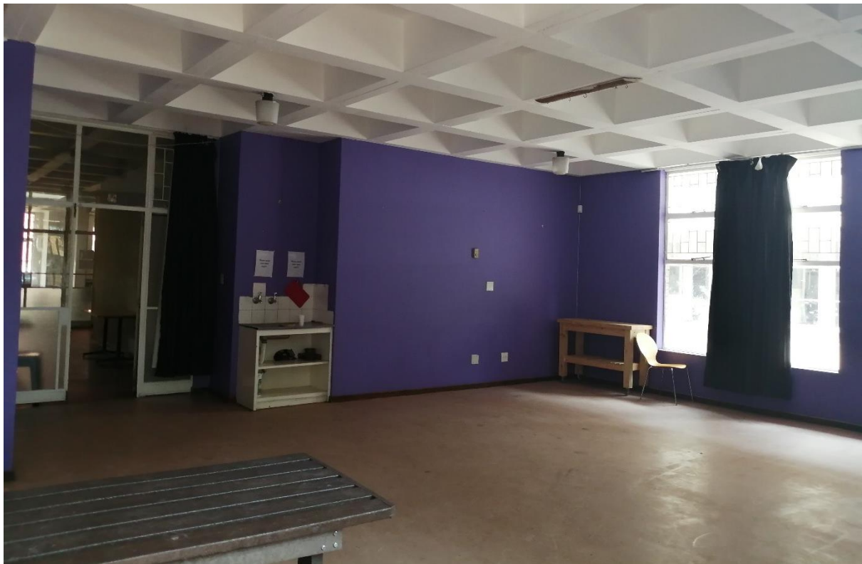
Figure 54: A standard adaptable classroom under renovation (Author, 2020).
