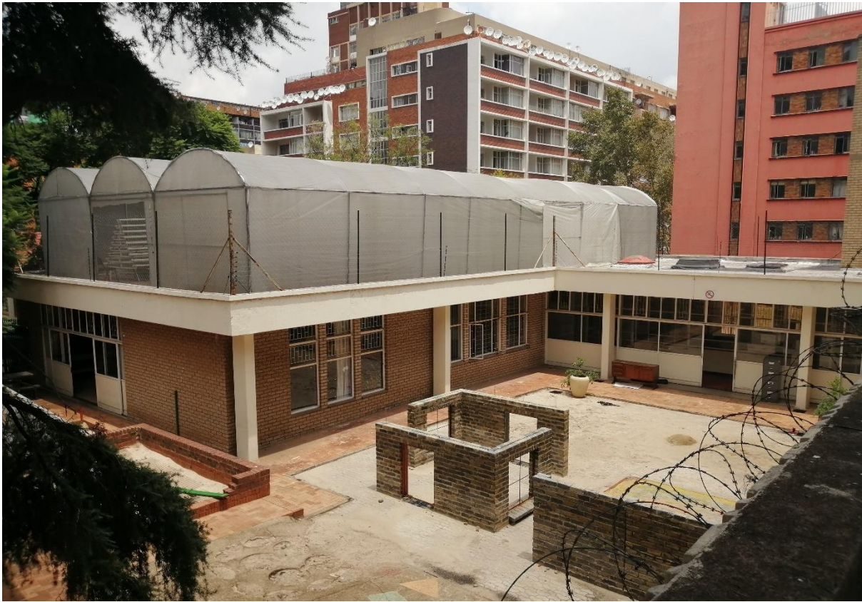
Figure 52: A central learning courtyard surrounded by classrooms as well as the roof greenhouse (Author, 2020).
