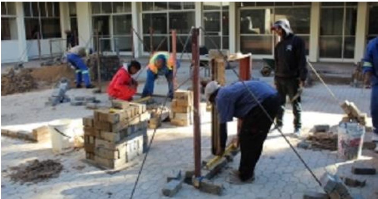
Figure 53: Skills development in the form of a bricklaying workshop (Outreach Foundation, 2019).
