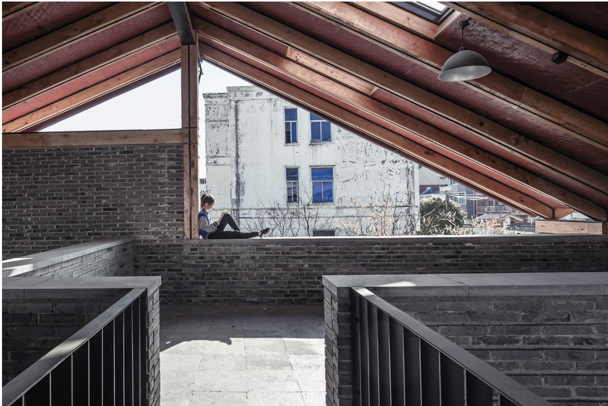
Figure 32: The community has the ability to adapt the building to suit their needs (ArchDaily, 2018).
