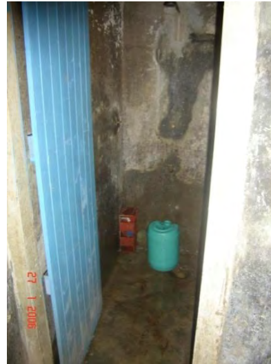
Photo 8. 26: Shower cubicle Source: Author
