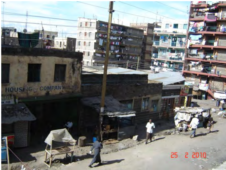
Photo 9. 11: Kiosks built along the pedestrian walkway forcing them onto the road. Source: Author
