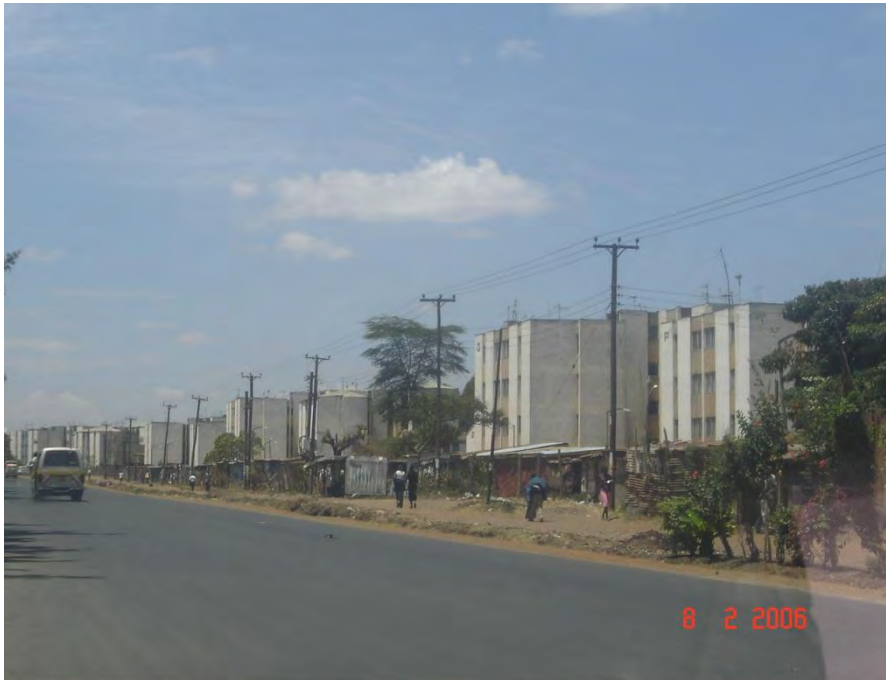
Photo: 5. 4 Huruma Estate, Nairobi City Council rental housing Source: Author
