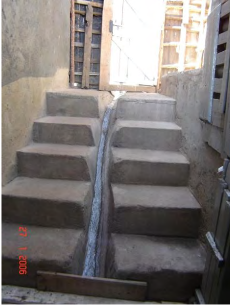
Photo 8. 5: Surface drainage in upgraded section Source: Author
