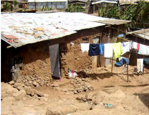
Photo 8. 18: Wattle and daub structure prior to upgrading. Source: Author
