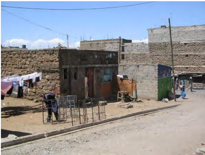
Photo 9. 8: Steel windows fabrication by the roadside. Source: Author
