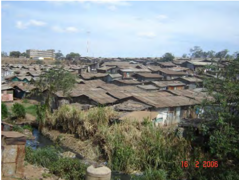
Photo 7. 1: Rusty metal sheet walls and corrugated iron sheet roofs reused after salvaging from previous fires in the area.
