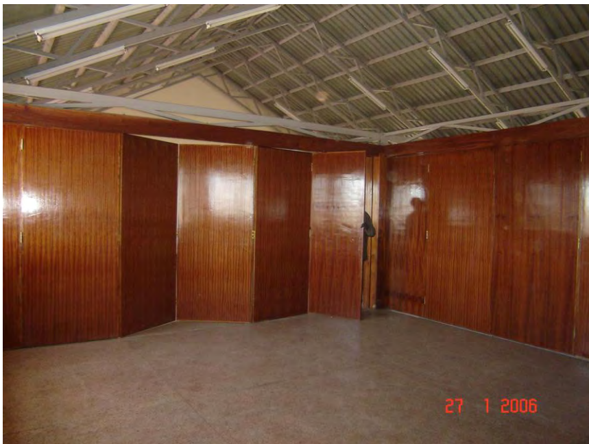
Photo 8. 12: Multipurpose hall above Baraka Medical Centre with folding partitions for multiple use. Source: Author
