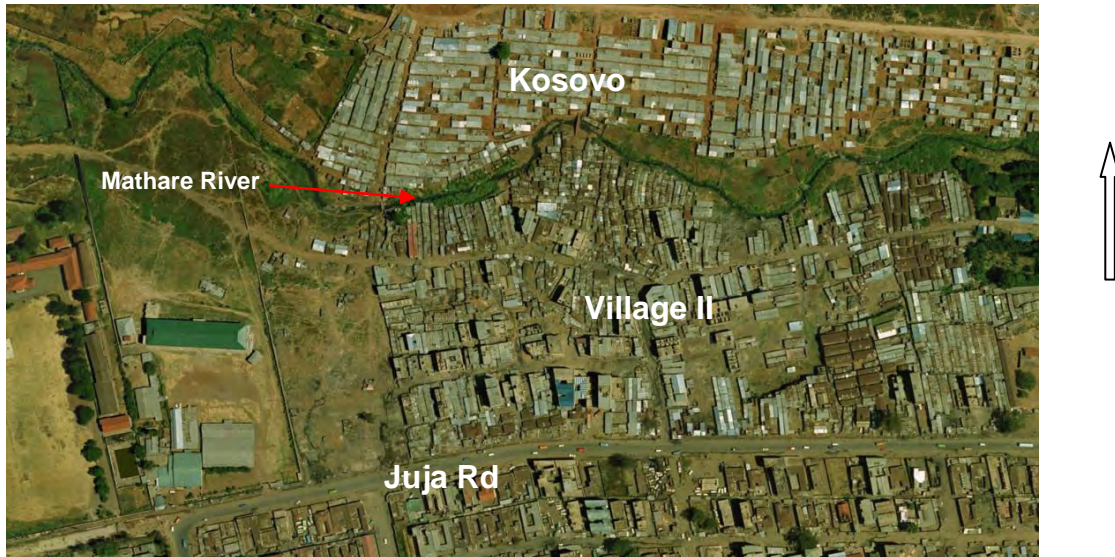
Figure 6. 13: Aerial view of Village II. Section demolished in recent years is shown on the left of the photo.
