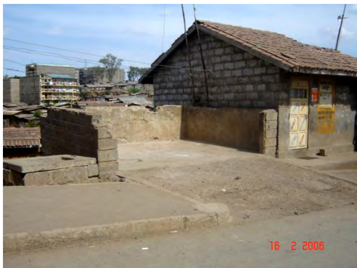
Photo 8. 13: Abandoned garbage collection point
