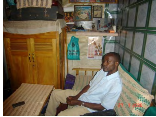
Photo 8. 23: Polyvinyl material used as wall lining on stabilized earth walls in improved housing
