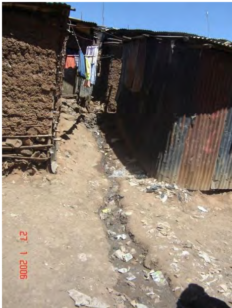
Photo 8. 3:Unpaved drainage prior to upgrading Source: Author
