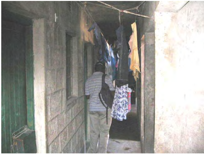
Photo 9. 13: A dark and narrow corridor within the above building with wet clothes hanging for drying. Source: Author
