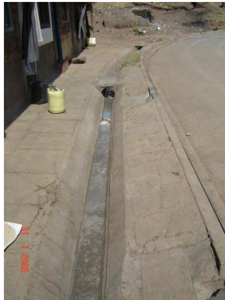
Photo 8. 4: Paved drainage after upgrading Source: Author
