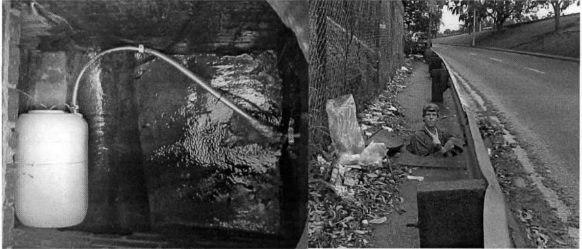
Plate 4-8: Installation set up for the N3 Highway and manhole entrance
