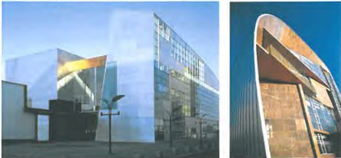
(Plate 6.14 & 6.15: The copper panels and zinc side-cladding on the curved wall is seen above. Aluminium sanded sheets on the straight exterior side walls reflect the sunlight. Source: www.helsinkiinstyle.fi , aedesign.wordpress.com )
