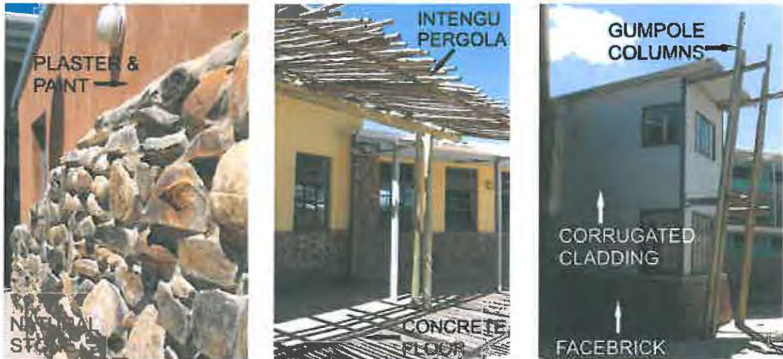
(Plate 7.38, 7.39 & 7.40: Photographs above illustrate the variety of materials used throughout the school, enhancing its tactile qualities. Source: Author)
