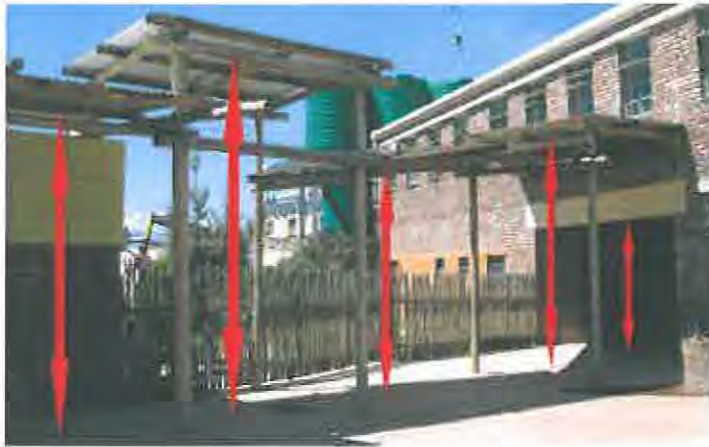
(Plate 7.42: Roof level changes break down the scale of the building. Source: Author)
