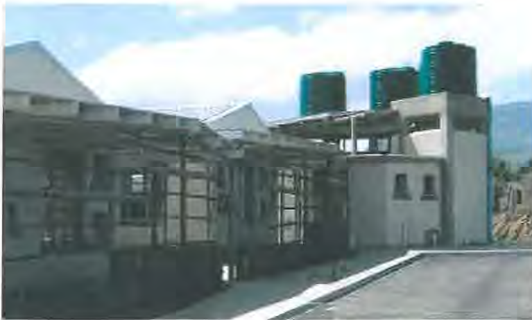
(Plate 7.53: View of the numerous Jo-Jo tanks used as an architectural feature. Here, they give the building height and are a beacon in the community. Source: East Coast Architects, 2011)
