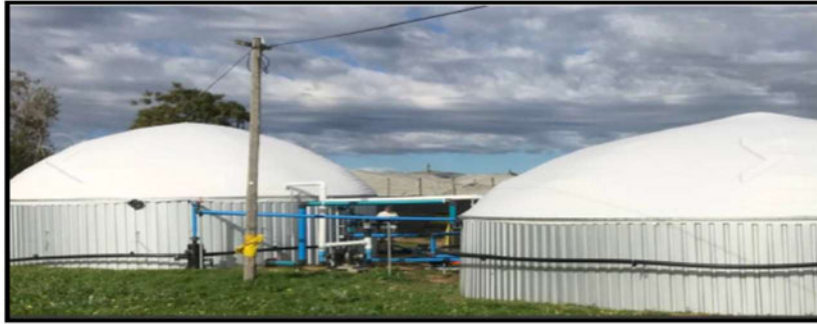
Figure 11: Biogas Demo Plant Installed in the Western Cape, South Africa (2018) [17].
