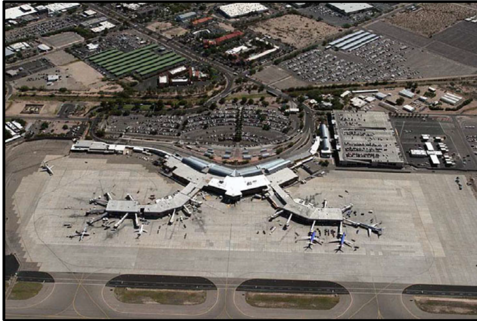
Figure 4: Project in progress – Tucson Airport application of the ceramic based thermal deflection paint [7]
