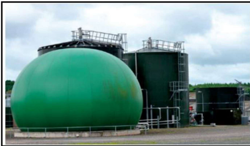
Figure 5: An on-Farm Anaerobic Digester Plant Showing the Gas Storage Tank and Digesters [2].
