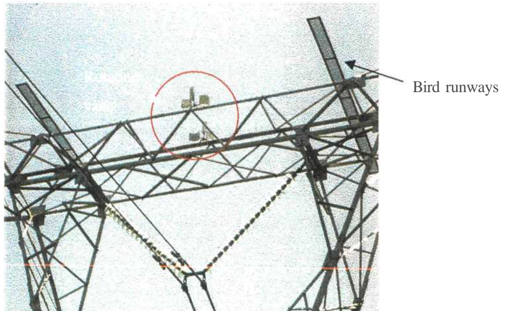
Figure 39. Application of rotating vane bird guard with bird runways
