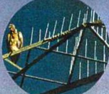
Vulture perched next to welded rod bird guards
