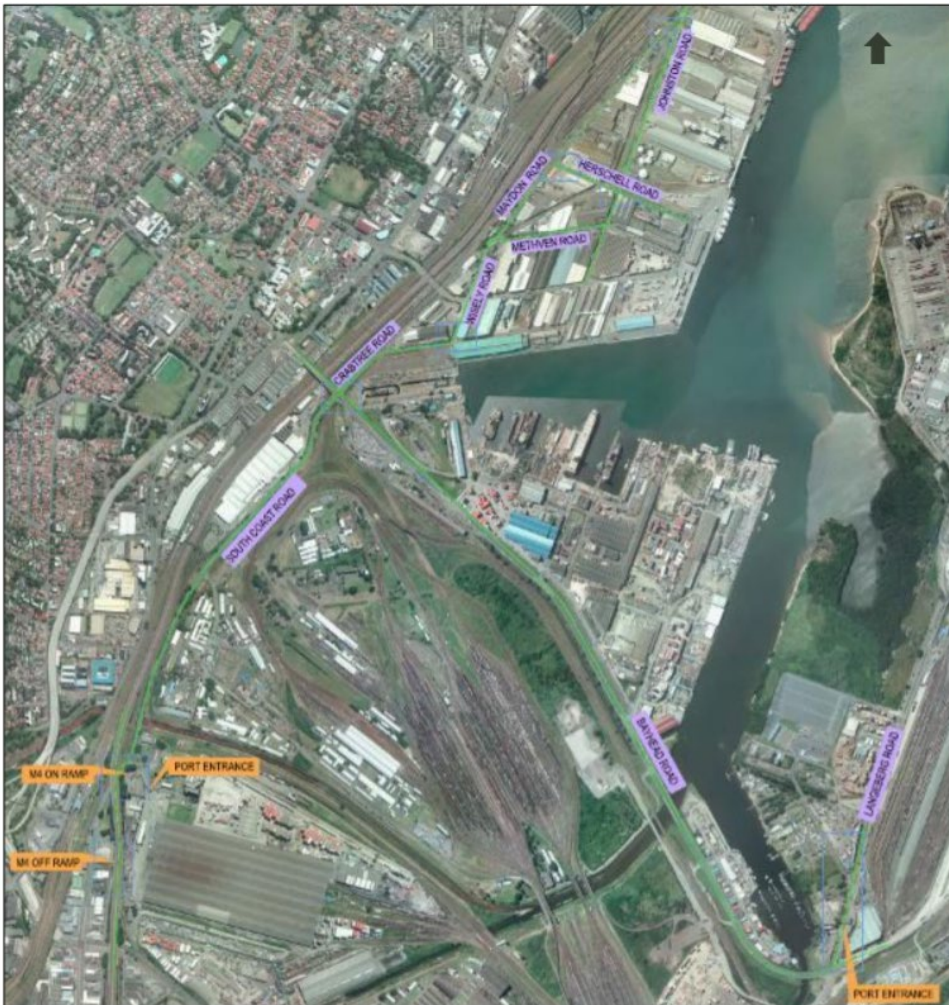
Figure 2. 4 Roads in the South end of the Port of Durban
