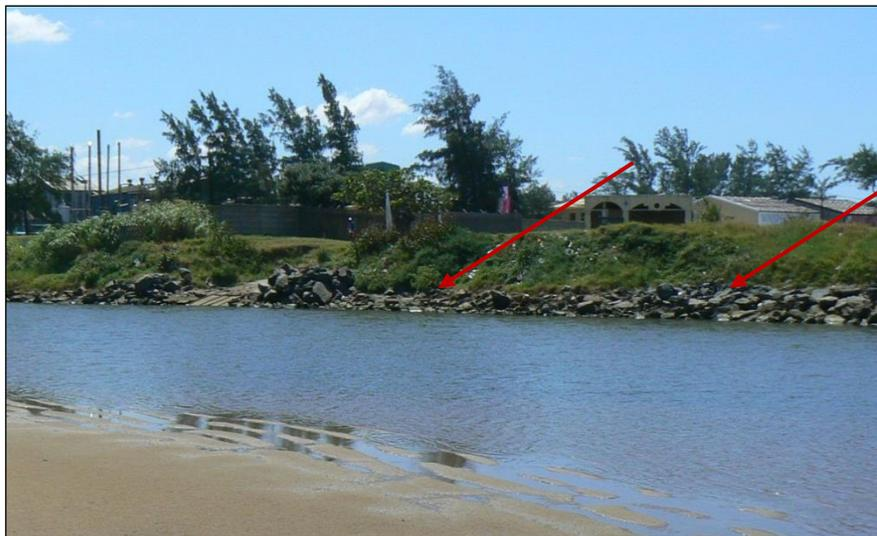
**Plate 2.3** Remnants of the gabion baskets used to artificially stabilize the northern bank of the estuary
