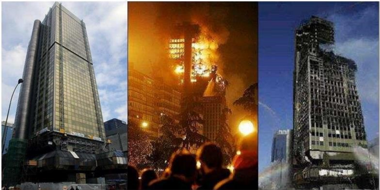
Figure 2.3: Windsor Building Fire (Qin, 2016)
