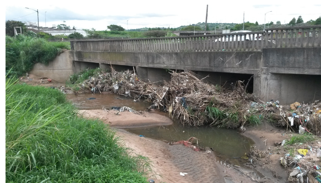
[1] - 29°48'20.0"S, 30°57'54.37"E Varsity Drive Bridge has become an accumulation point for waste.
