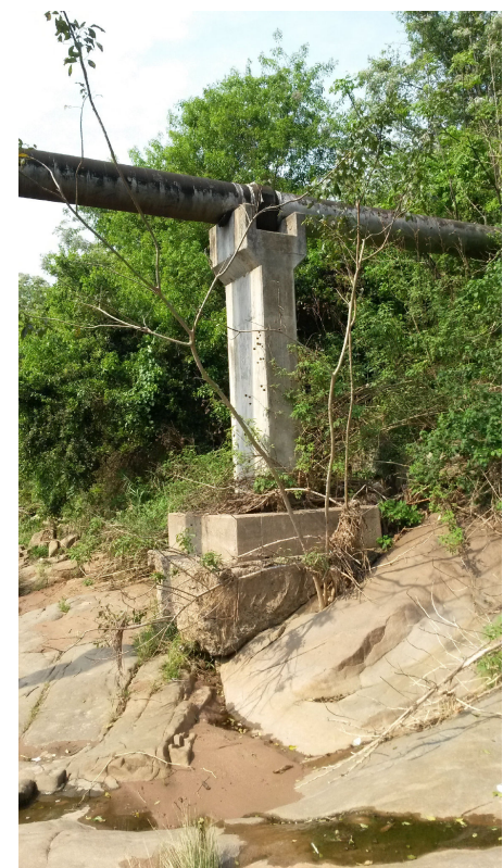
[2] - 29°49'29.4"S, 30°56'58.5"E Sewer line running across the Palmiet River.
