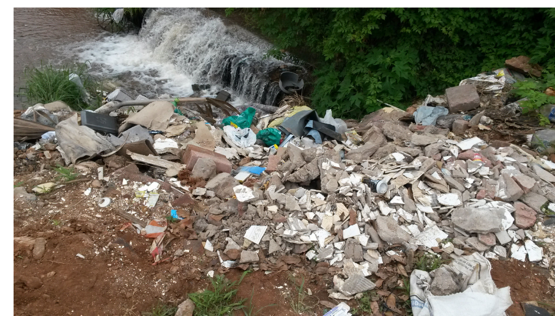
[3] - 29°48'16.8"S, 30°57'56.0"E Contractors dump building rubble at the Quarry Road Informal Settlement.
