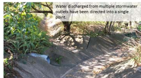
Figure D-15: [3.5 - 5] Section 2 New Germany Nature Reserve (Unit 4).
