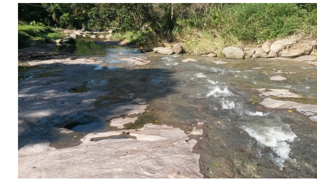
[4] - 29°49'11.9"S, 30°53'36.0"E Riverbed has been scoured down to bedrock
