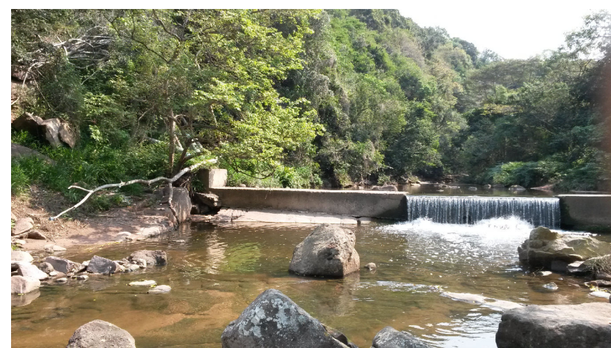
[3] - 29°49'30.4"S, 30°55'59.6"E Weir constructed across the river channel.
