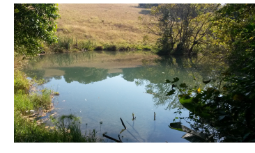
[2] - 29°48'46.0"S, 30°53'27.3"E Hammerkop Dam wall compromised
