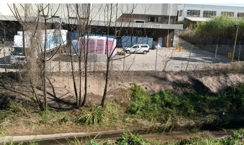
[5] - 29°48'15.3"S, 30°52'13.9"E Palmiet River bank has been cemented
