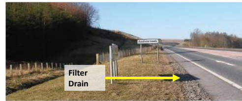
Figure 2-8: Example of a filter drain implemented along a road (Source: CIRIA, 2015a).
