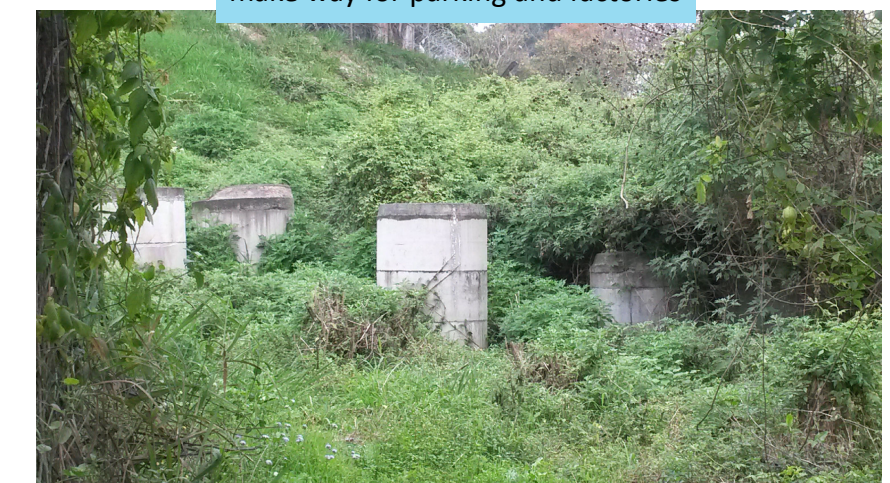
[9] - 29°48'52.9"S, 30°52'51.6"E Numerous sewer manholes in the riparian zone of the Palmiet River
