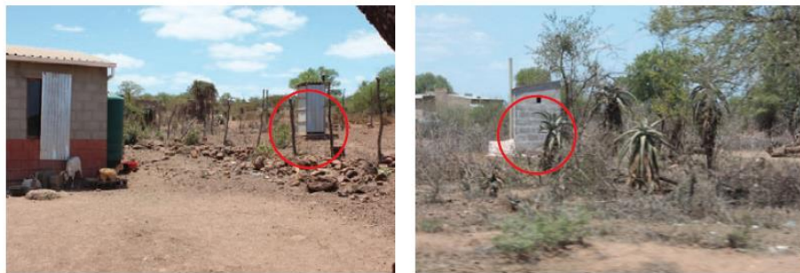
Photo 2 The two types of VIP-toilets common in the community. The one on the left is made out of corrugated iron, and the one on the right is made out of bricks.
